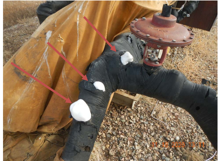
Photo 3. Ice from high pressure leak at separator.
