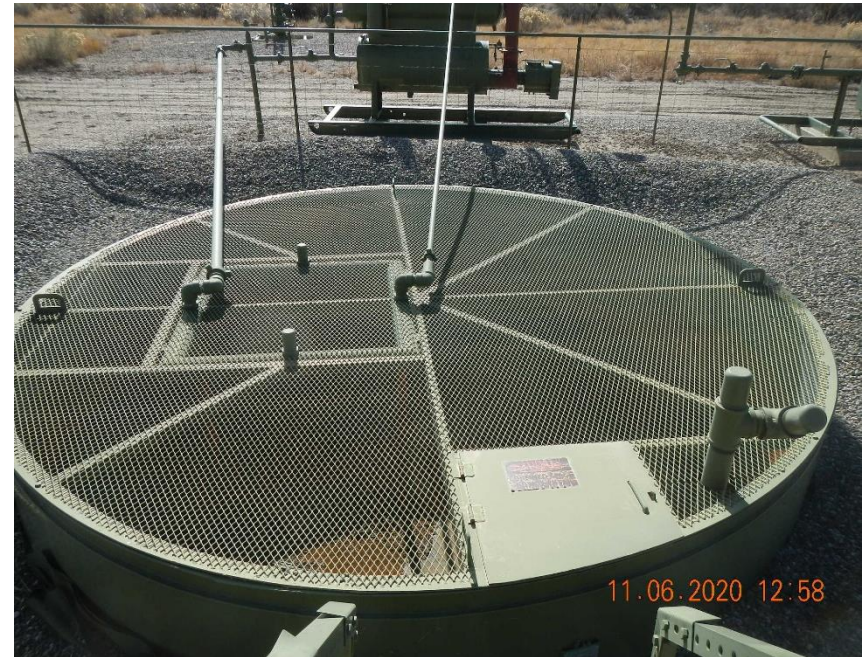
Open topped vessel has 120 bbl. capacity stamped on side.
