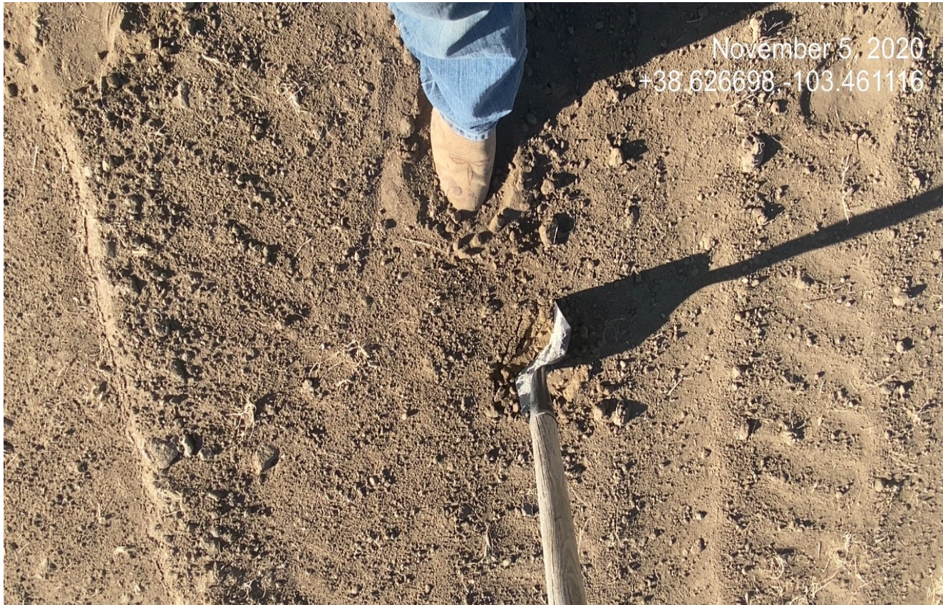
Photo 6. The topsoil pile has been tracked but is not sufficient to stabilize and maintain the topsoil pile. The topsoil is susceptible to erosion.
