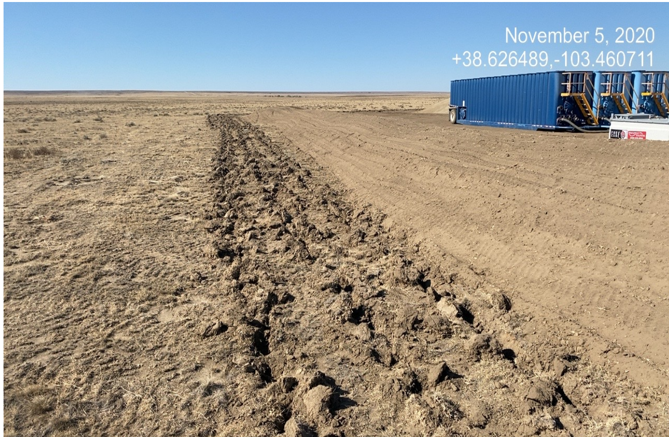
Photo 4. Facing northwest. Surface roughening has been performed around the location and a topsoil berm is placed around the perimeter of the location.
