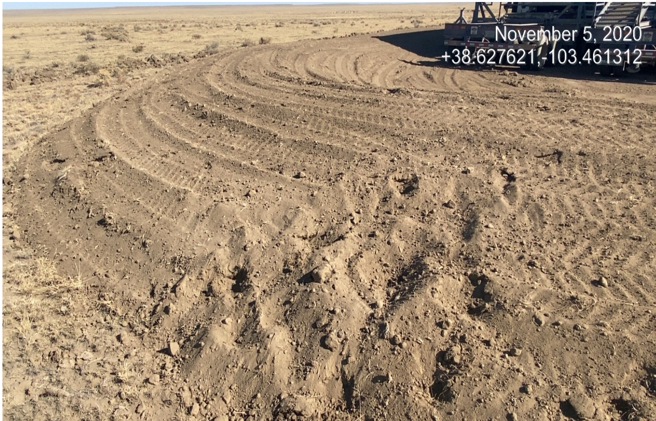
Photo 10. There is cattle tracks on the topsoil pile showing that the topsoil is loose and not stabilized.
