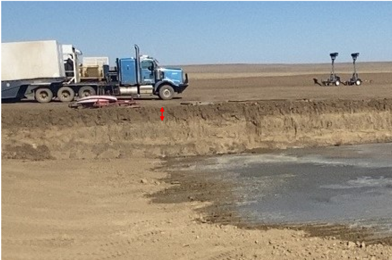
Photo 9. This photo is zoomed in to show the soil horizon in the excavated pit. There is a definitive color change in the soil indicating soil horizons. Additional topsoil (dark horizon) should have been salvaged.
