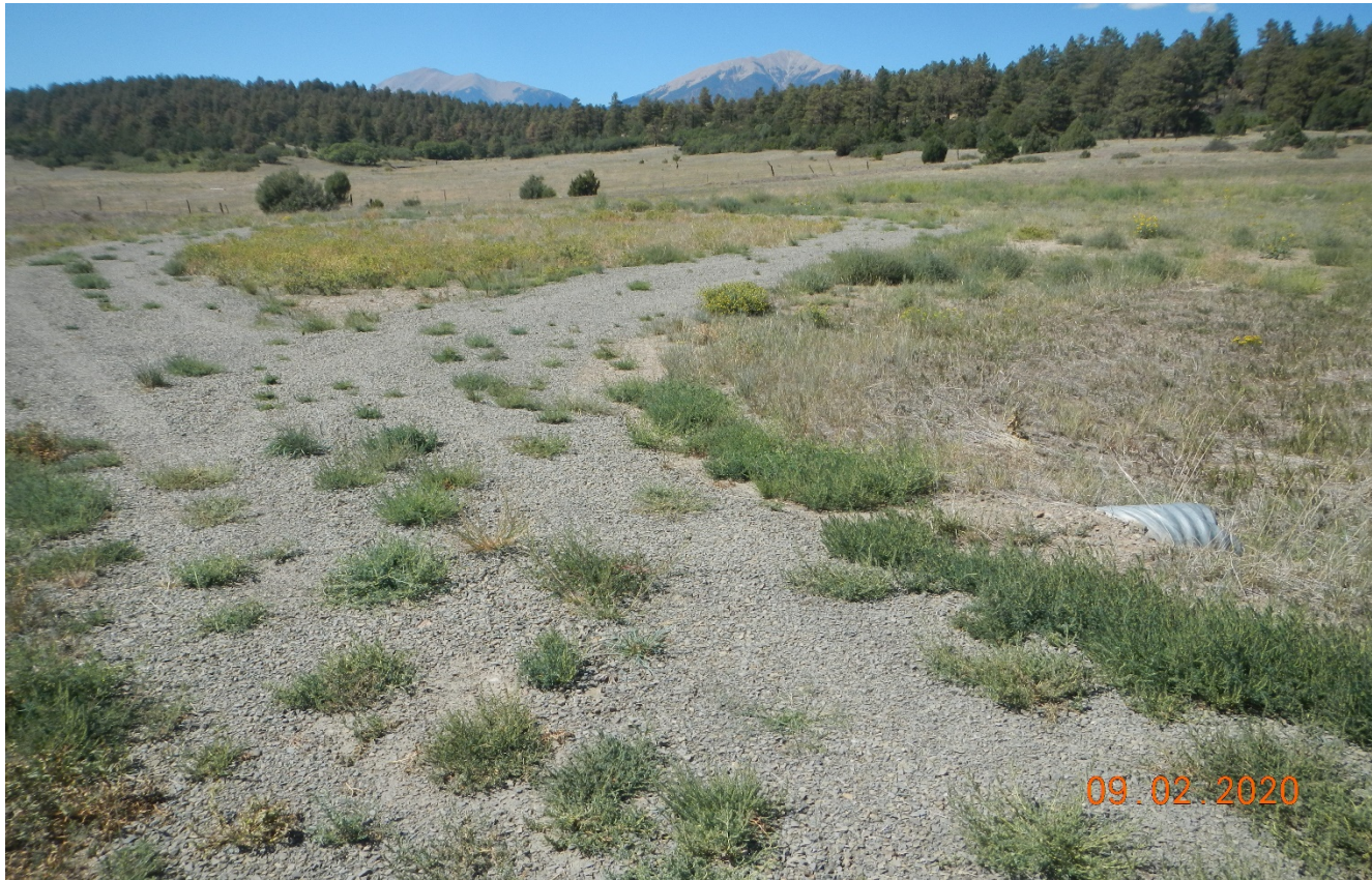
Photo 3. Facing northwest toward the location. Gravel remains around the location and there is a culvert that has not been removed. Location has not been reclaimed.
