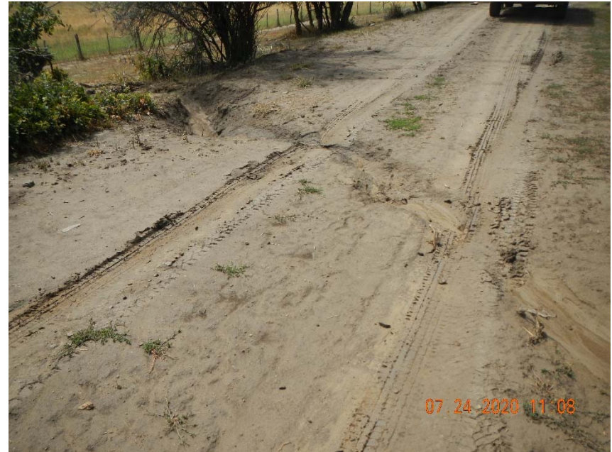
Photo 4. Sediment migration down and off access road.
