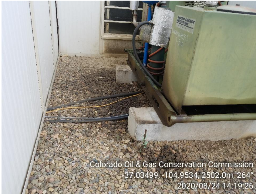
PHOTO 3: AREA OF IMPACTED SOIL AROUND DRIVEHEAD ENGINE SKID. Conduct maintenance on equipment, cleanup IMPACTED SOIL and review self inspection processes. CA DATE 11-24-20.
