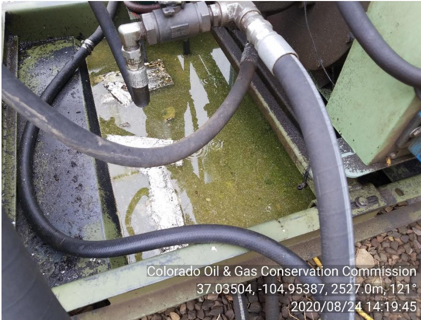
PHOTO 5: OILY FLUID STORED IN ENGINE SKID.
