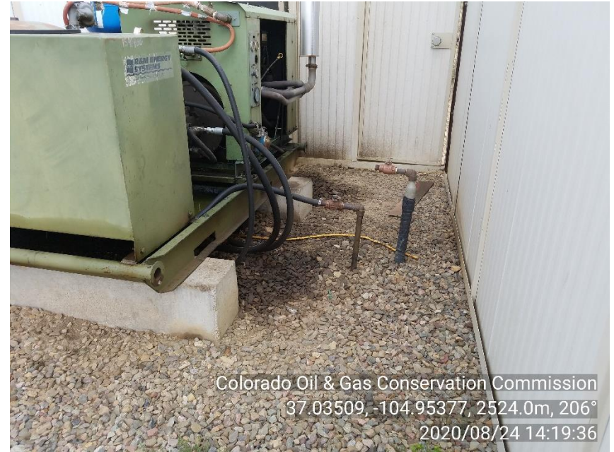
PHOTO 4: ANOTHER IMAGE OF IMPACTED SOIL AROUND ENGINE SKID.
