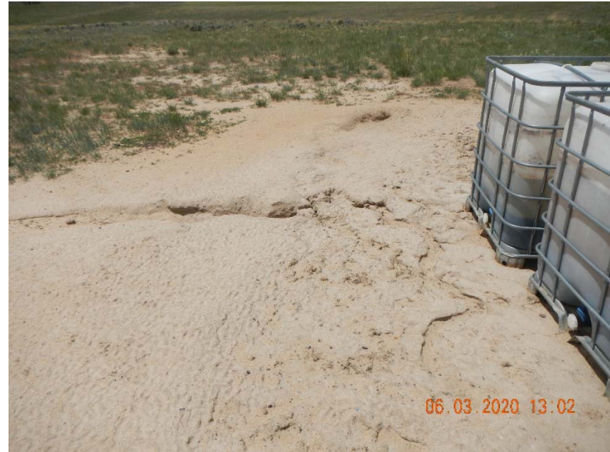
Photo 8. Erosion gully origin on east side of location. Containers without secondary containment.
