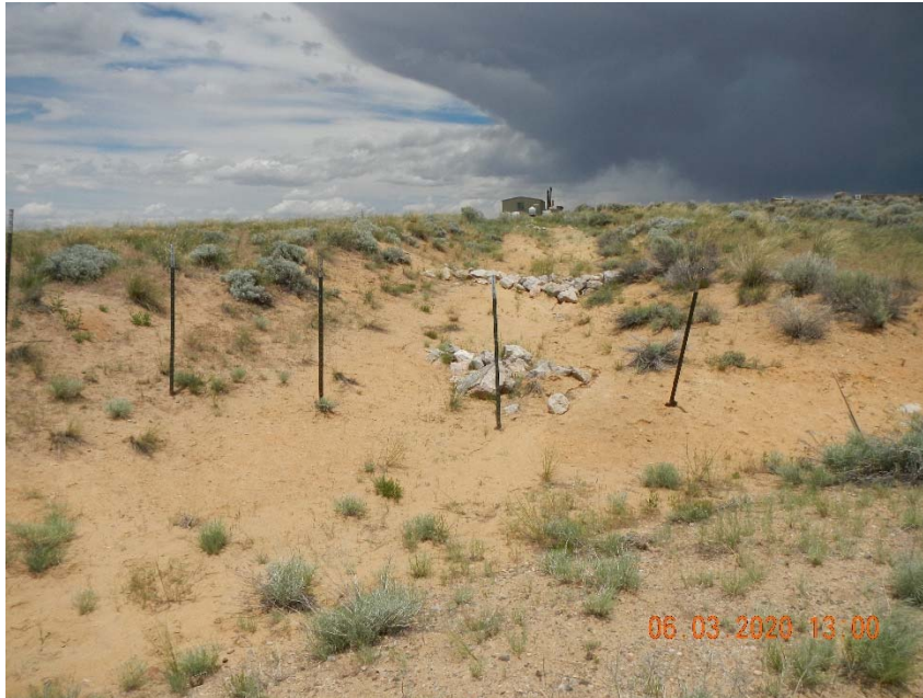
Photo 7. Erosion gully leaving location. Photo taken from access road looking towards location.
