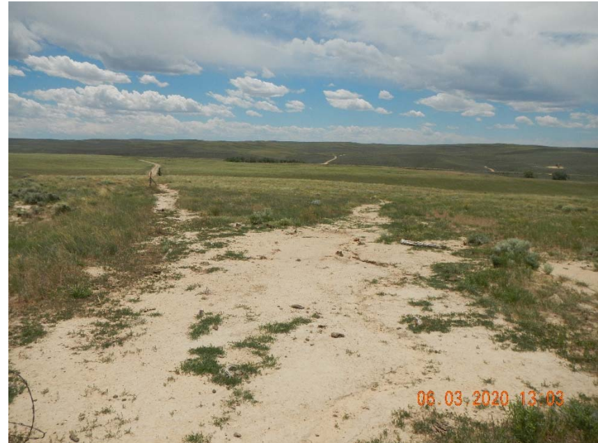
Photo 10. Erosion leaving location. Photo standing on location perimeter looking towards access road.
