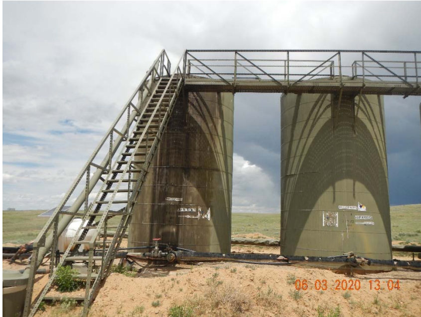
Photo 3. Incomplete or missing tank labels.
