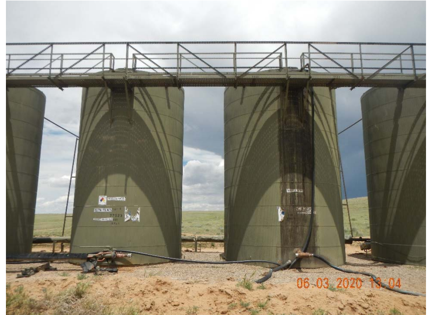
Photo 4. Incomplete or missing tank labels.
