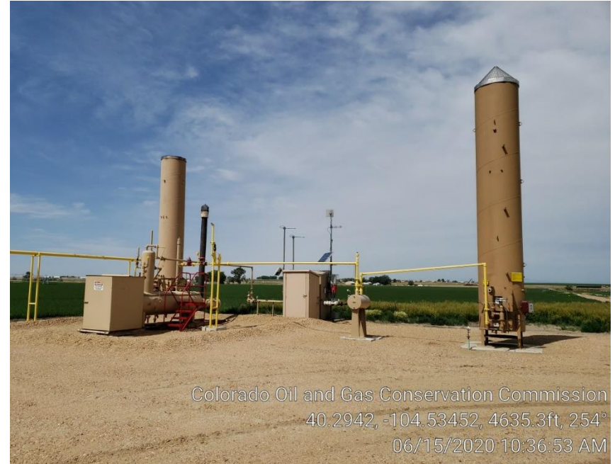
Photo #2 Separator, ECDs & Meter Runs
