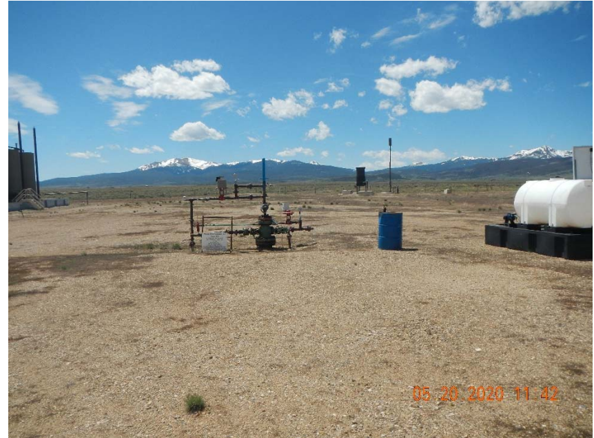
Photo 2. Two unlabeled containers at wellhead. Blue drum without secondary containment.
