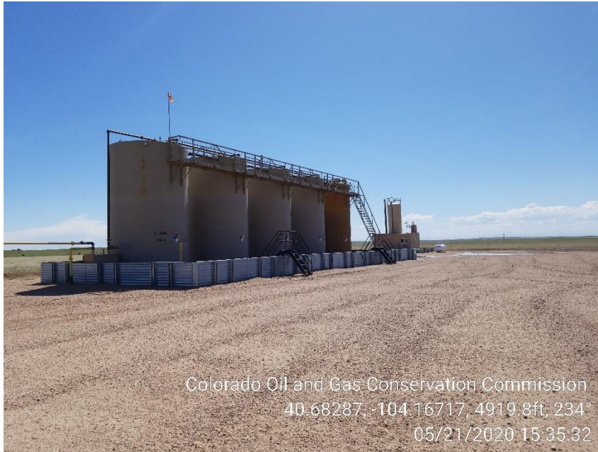
Photo 1 – Tank Battery
