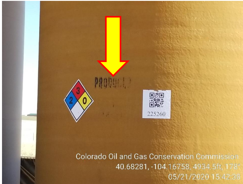
Photo 5 – Produced Water Tank missing Capacity and Content is fading
