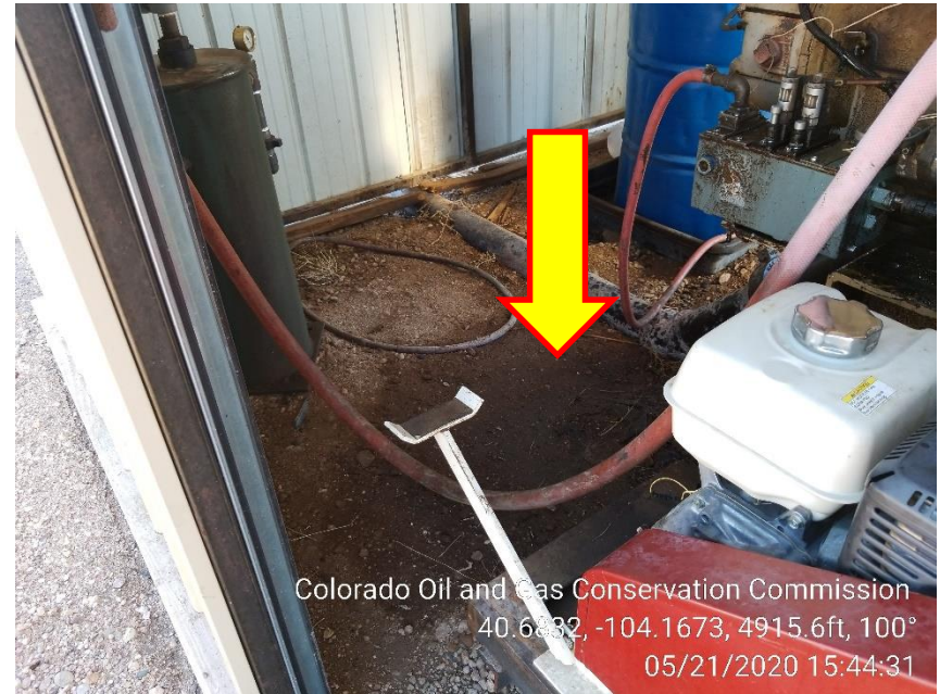
Photo 6 – Stained Soil at Gas Engine
