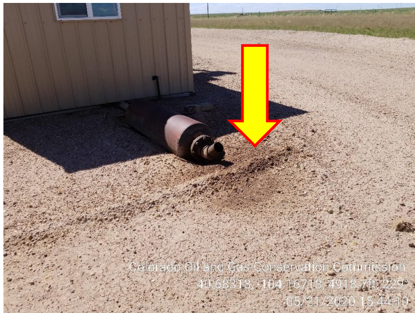
Photo 7 – Stained Soil at Exhaust
