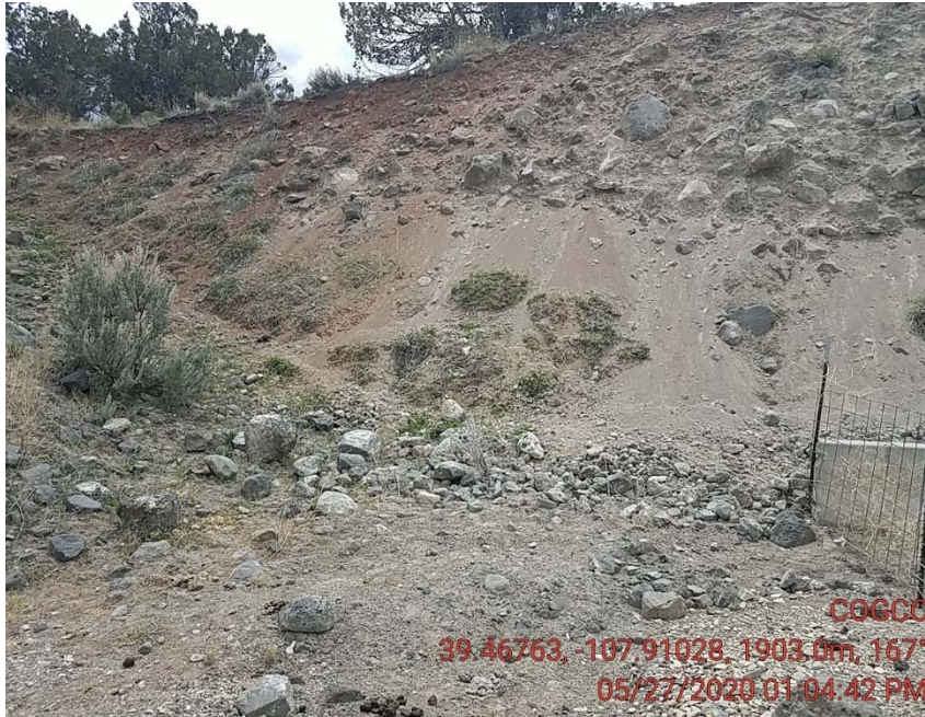
Slope sluffing
