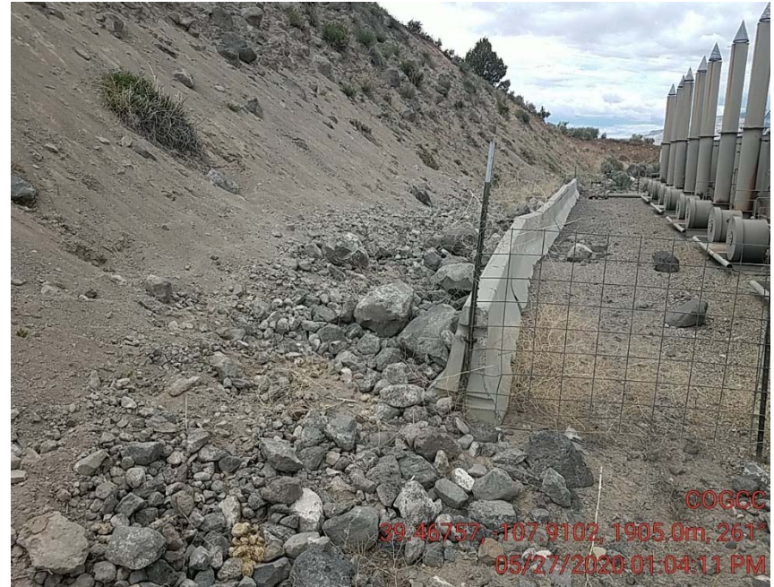
Slope sluffing
