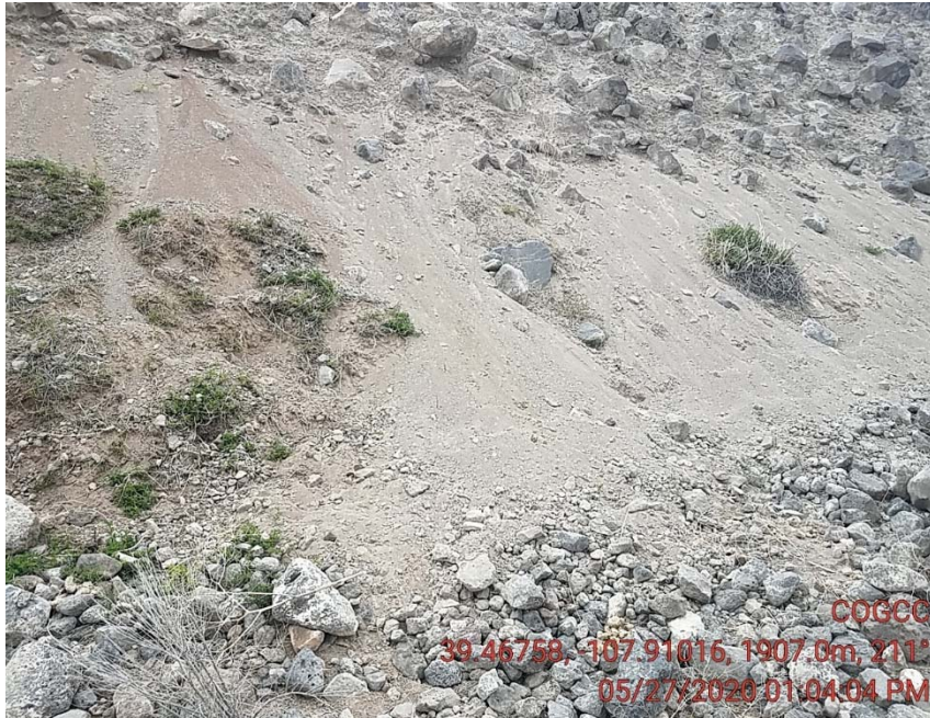
Slope sluffing
