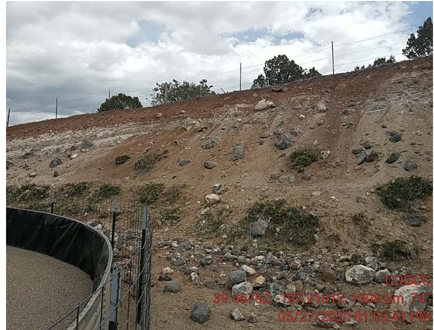
Slope sluffing
