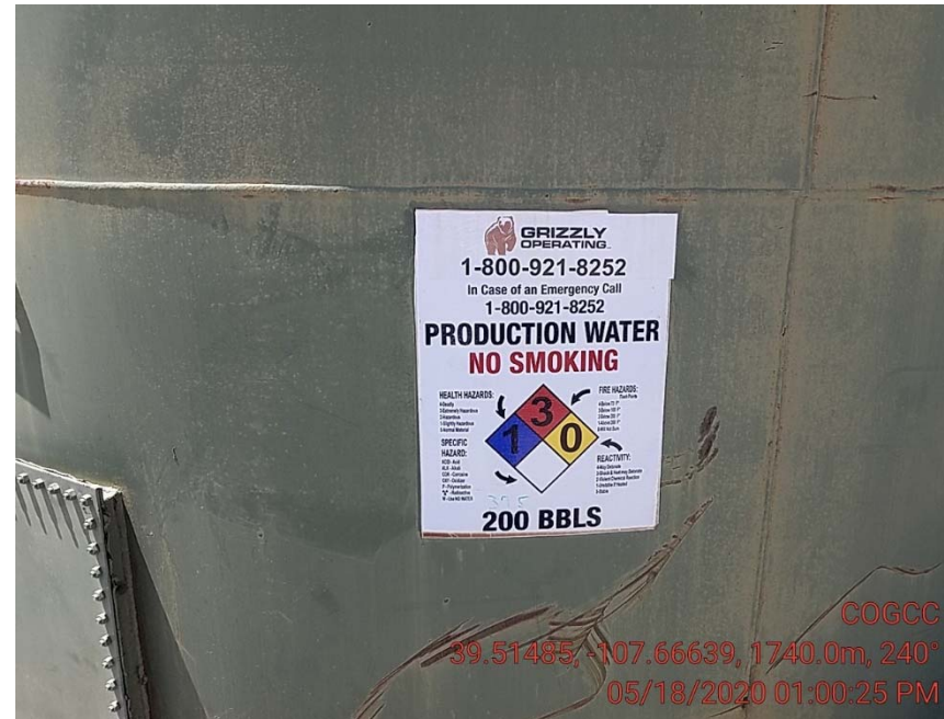
Tank label with incorrect quantity
