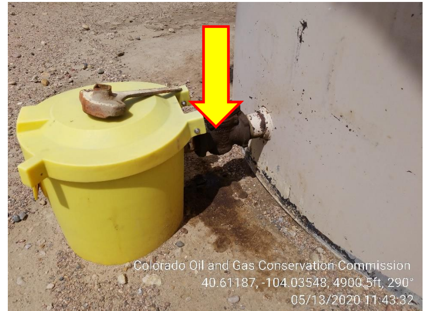
Photo 6 – Stained Soil at Loadline on West Tank
