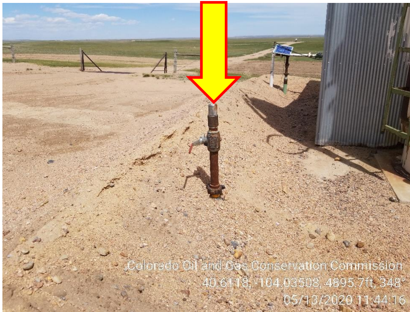
Photo 5 – Unmarked Riser at Heater Treater
