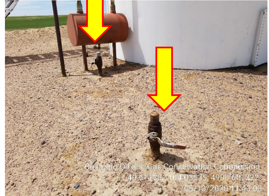
Photo 4 – Unmarked Risers at Tanks
