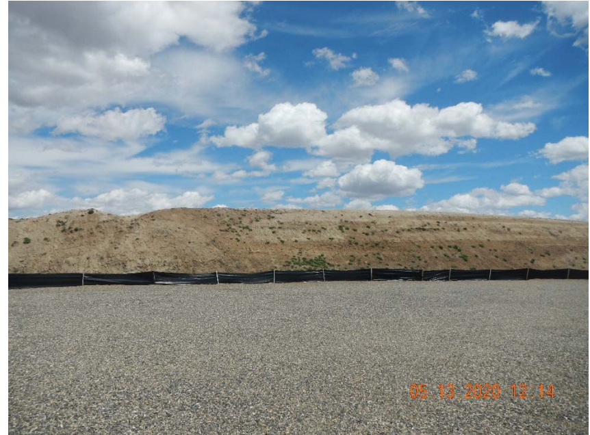
Photo 2. Erosion and weeds occurring on fill pile.
