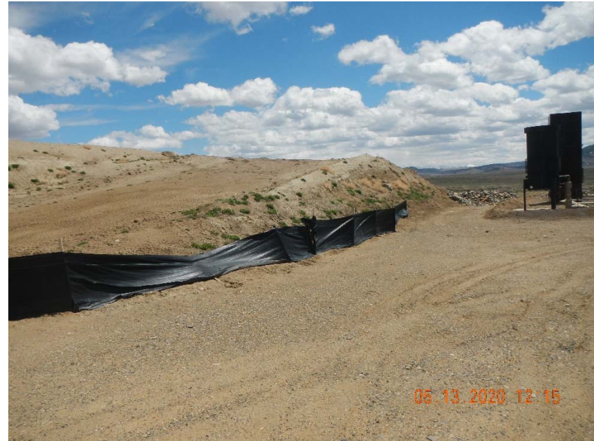
Photo 4. Erosion and weeds occurring on fill pile. Sediment moving under silt fence. Silt fence or other BMP not present on east end of fill pile.
