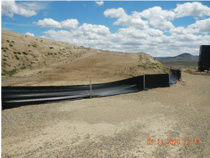
Photo 3. Erosion and weeds on fill pile. Sediment moving under silt fence.
