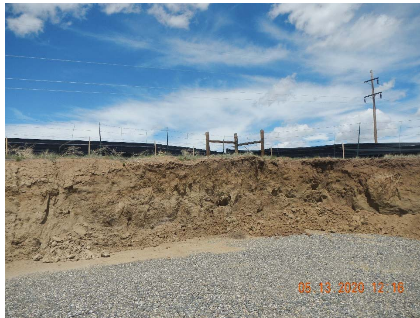
Photo 6. Erosion on cut slope.
