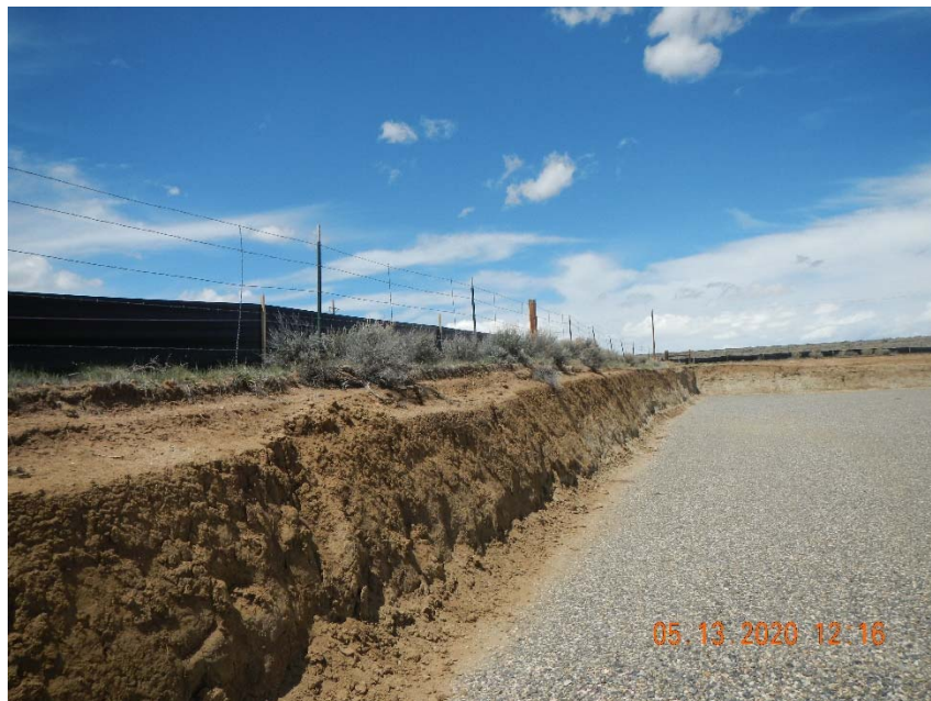
Photo 5. Erosion on cut slope.
