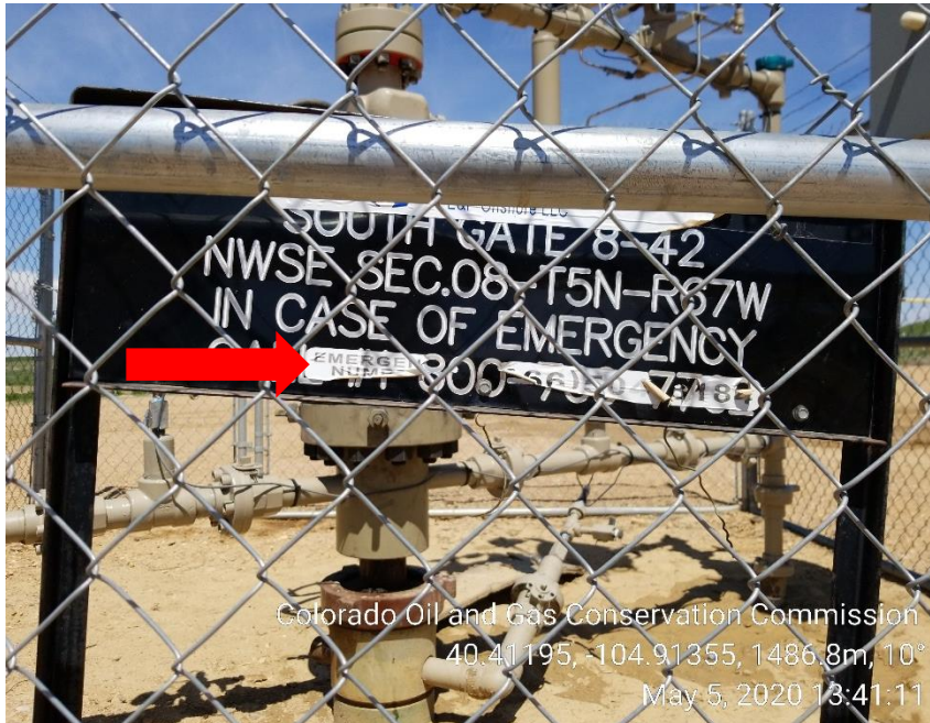
Photo 3: Wellhead Sign; missing emergency #
