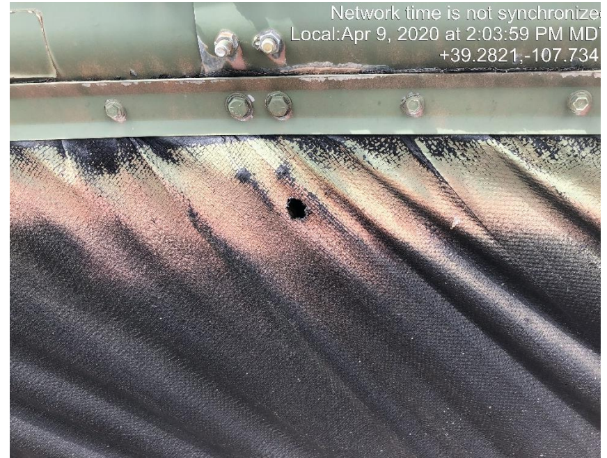
Photo #0946 Multiple holes in tank containment Liner.
