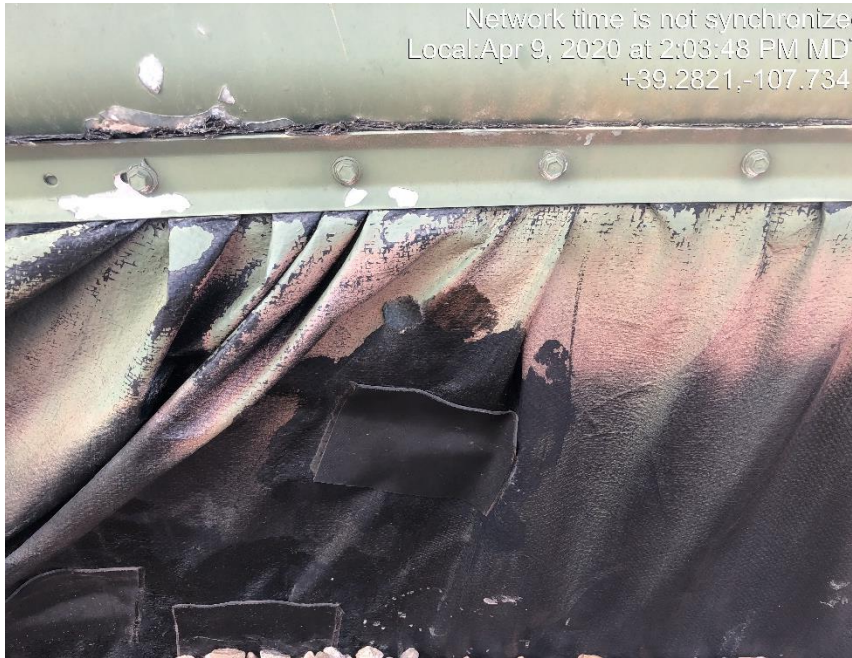
Photo #0945 Multiple holes in tank containment Liner.
