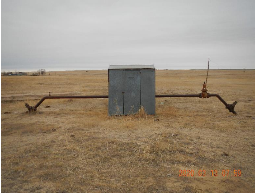
Photo 1: Gas meter run.
