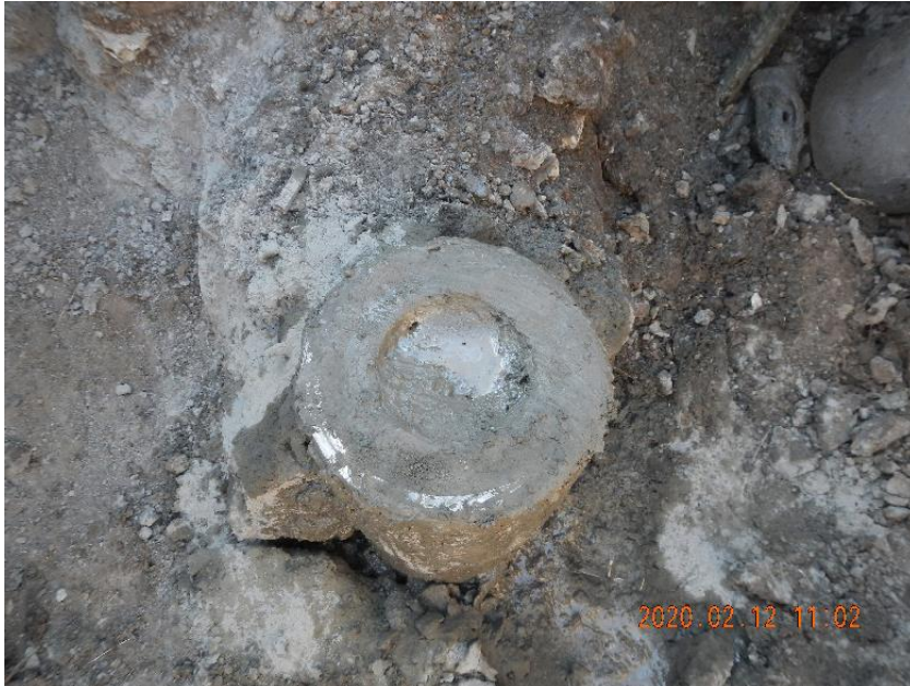
Photo 9: Cement topped off in surface casing.
