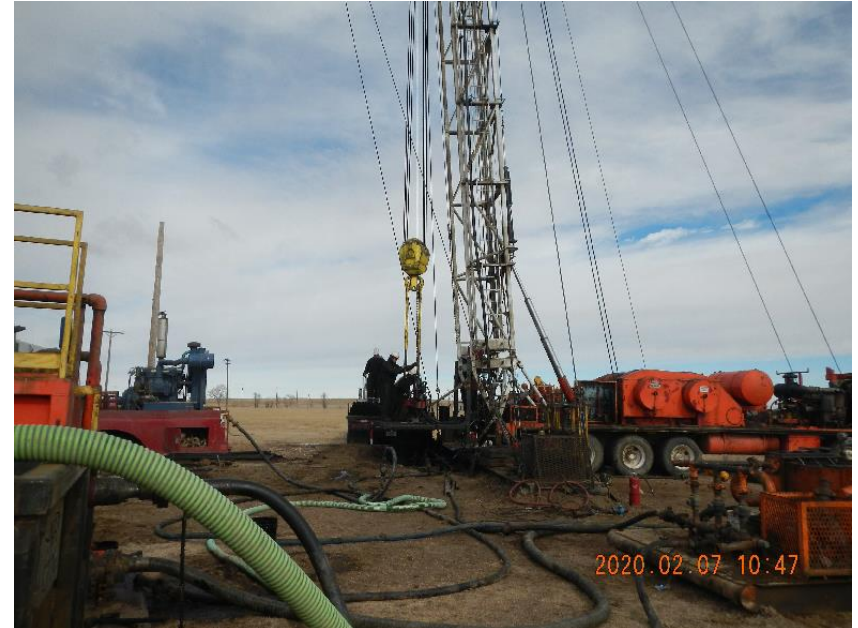
Photo 6: Equipment rigged into well to complete cement plug.
