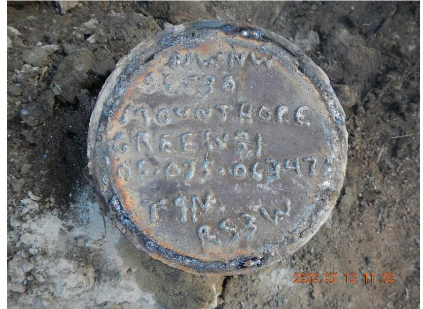
Photo 10: Marker plate welded onto surface casing.
