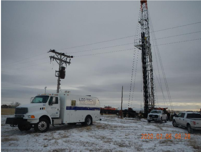
Photo 3: Wireline setting CIBP and running CBL on casing.
