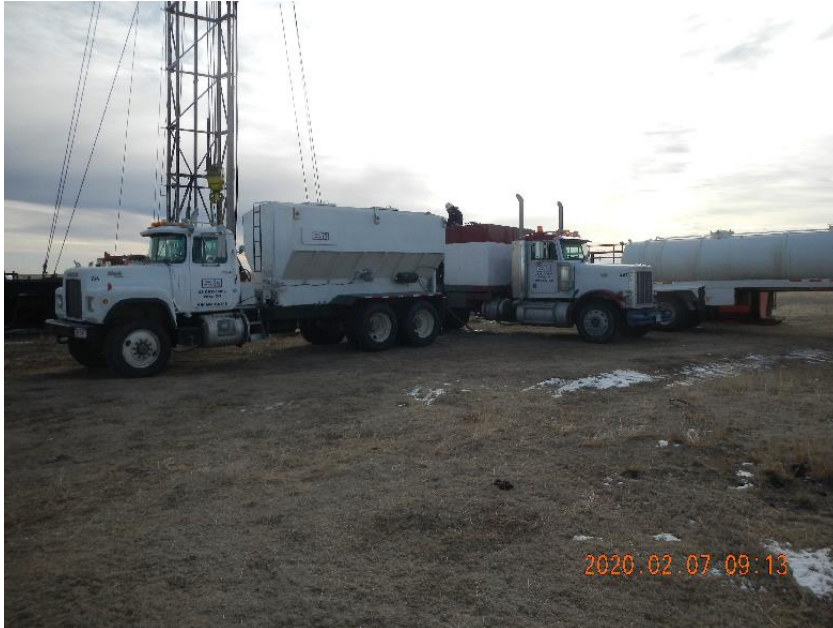
Photo 5: Cement crew on location to pump cement plugs.
