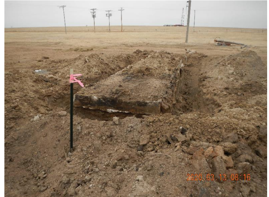
Photo 12: Marked surface casing. Cement pump jack base and power poles that need to be removed.
