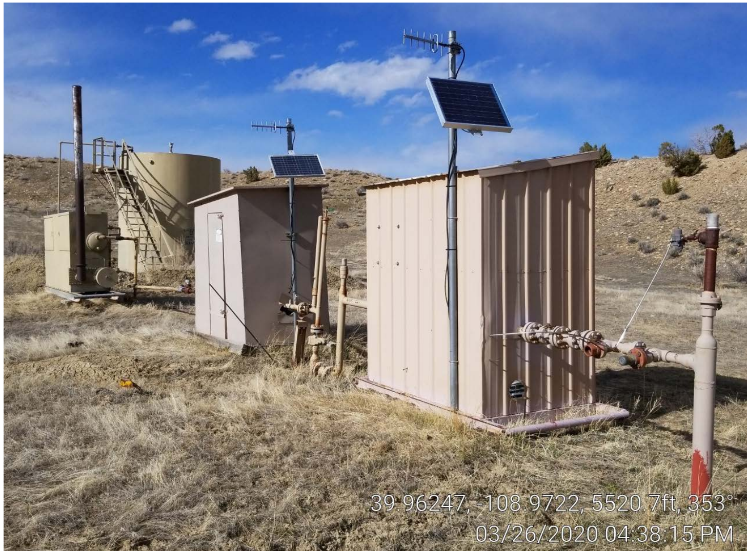
Photo 2. Meter buildings, separator, and tank.
