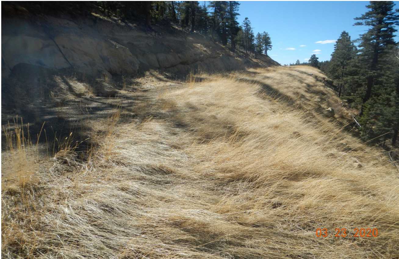
Photo 4. The vegetation is well established along the fill slope of the road.
