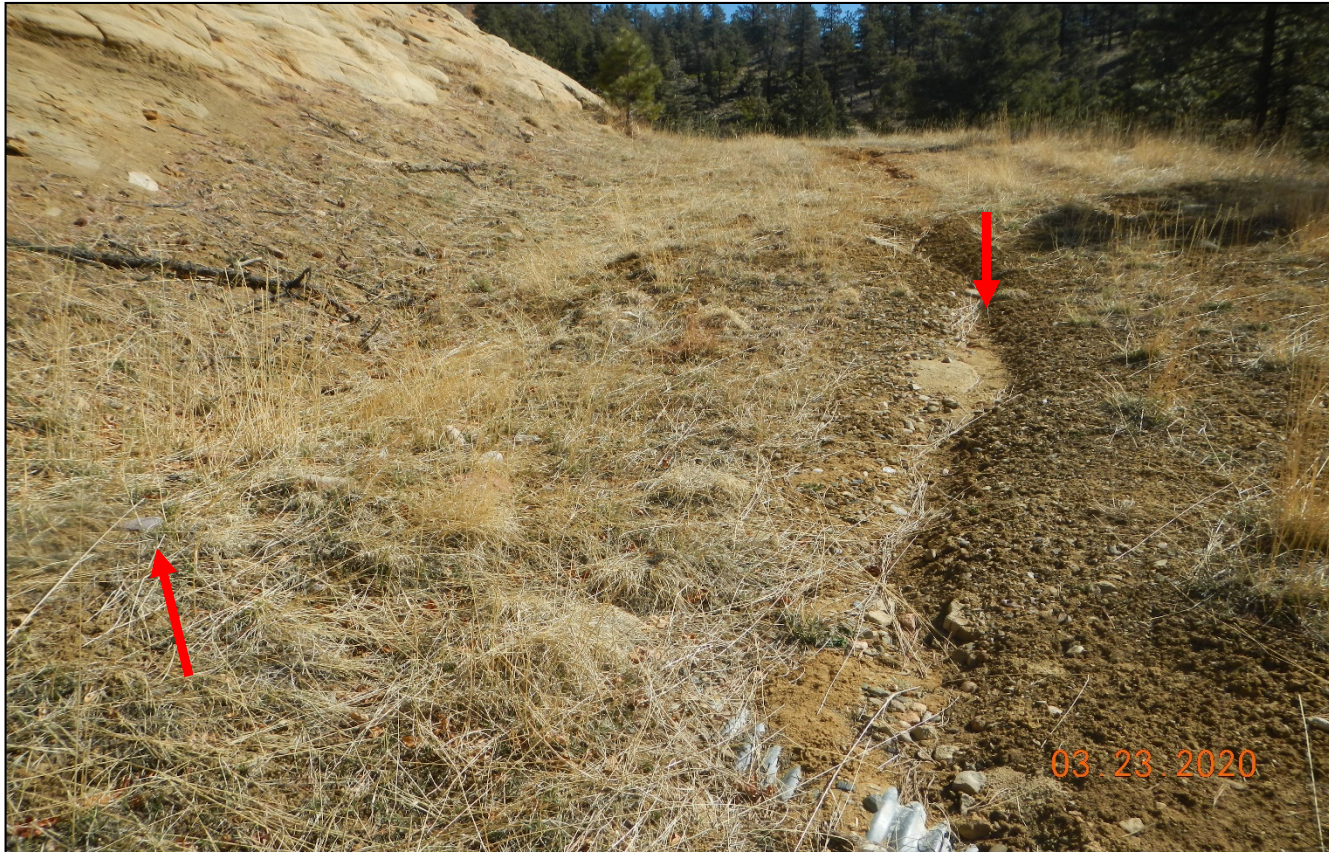
Photo 3. Another culvert further along the road is filled in with sediment and it appears stormwater is directed down the road.
