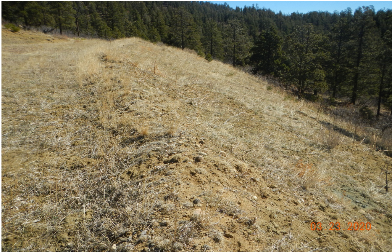
Photo 8. Facing east along the fill slope. Vegetation is well established along fill slope.
