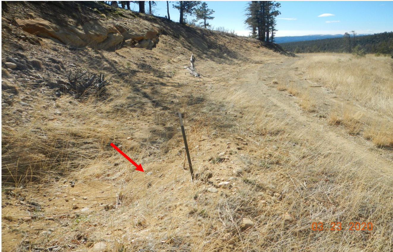
Photo 6. This culvert near the location is filled in with sediment.
