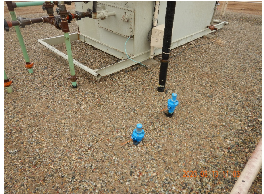
Photo #8 – Unused, marked, and plugged flowline risers located southwest of separators.
