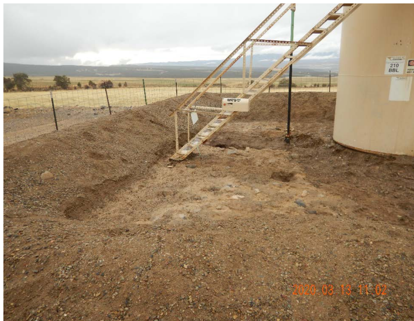
Photo #3 – View of south side of unlined earthen berm containment area.
