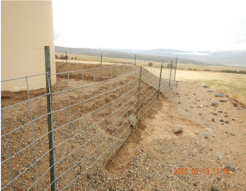
Photo #5 – Damaged section of earthen berm outside of north wall.
