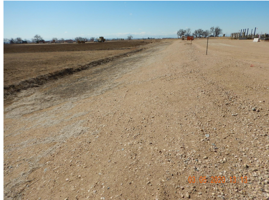
Photo 8. Photo taken from the southeastern production facility location, facing West. Photo illustrates a ditch and berm along the southern location that is directed to a stabilized outlet.
