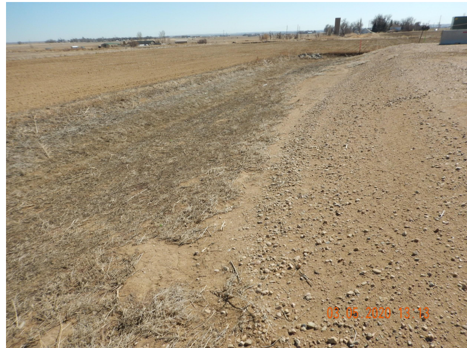
Photo 6. Photo taken from the eastern production facility location, facing South. Photo illustrates a retention area with a stabilized outlet (southeastern corner).
