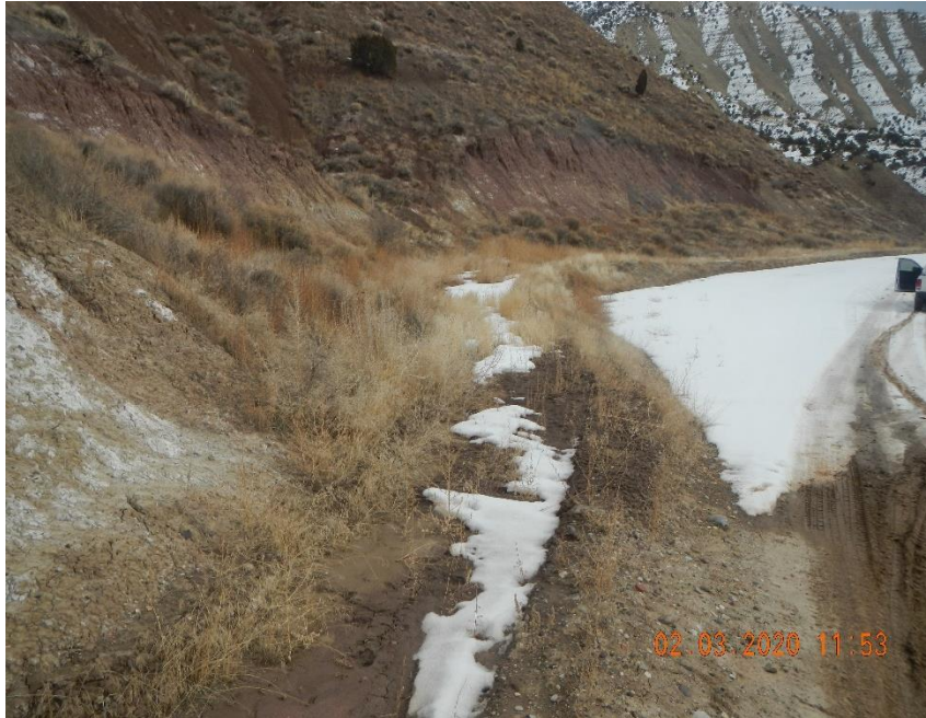
Sediment build up in ditch.
