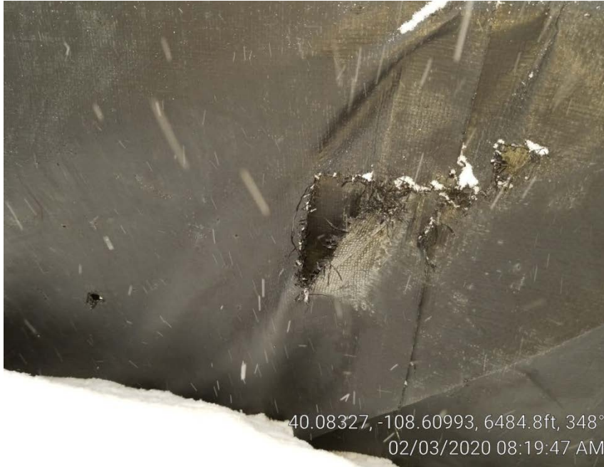
Photo 10. Tank secondary containment liner on 2-3-2020.
