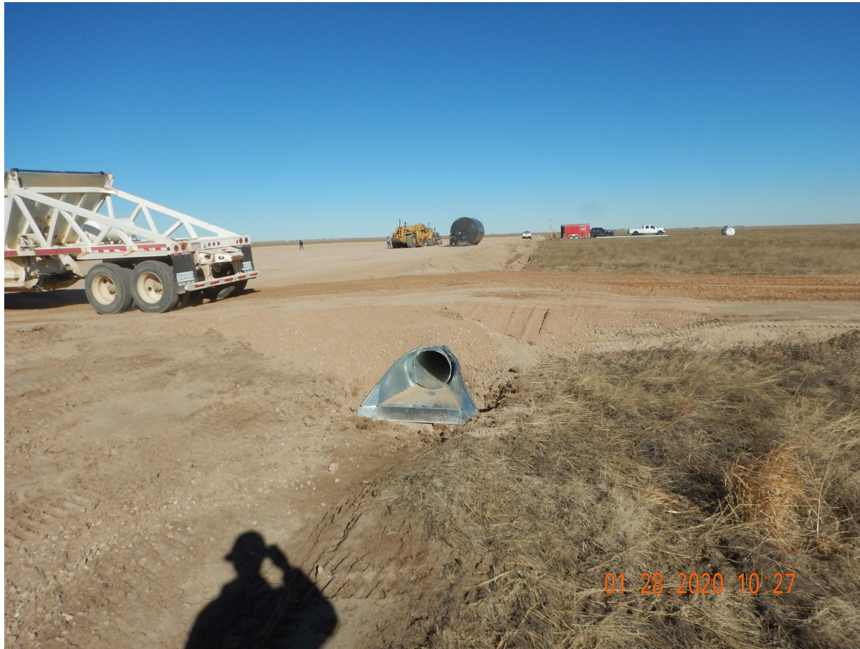
Photo 9. Photo taken from the southeastern perimeter of location, facing North. Photo illustrates a culvert installed in conjunction with the ditch BMP which is directed to a sediment trap.
