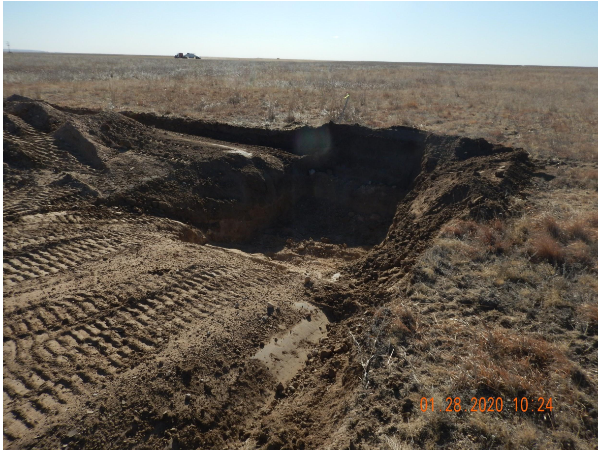
Photo 6. Photo taken from the southwestern perimeter of location, facing South. Photo illustrates a sediment trap in-process of being installed.
