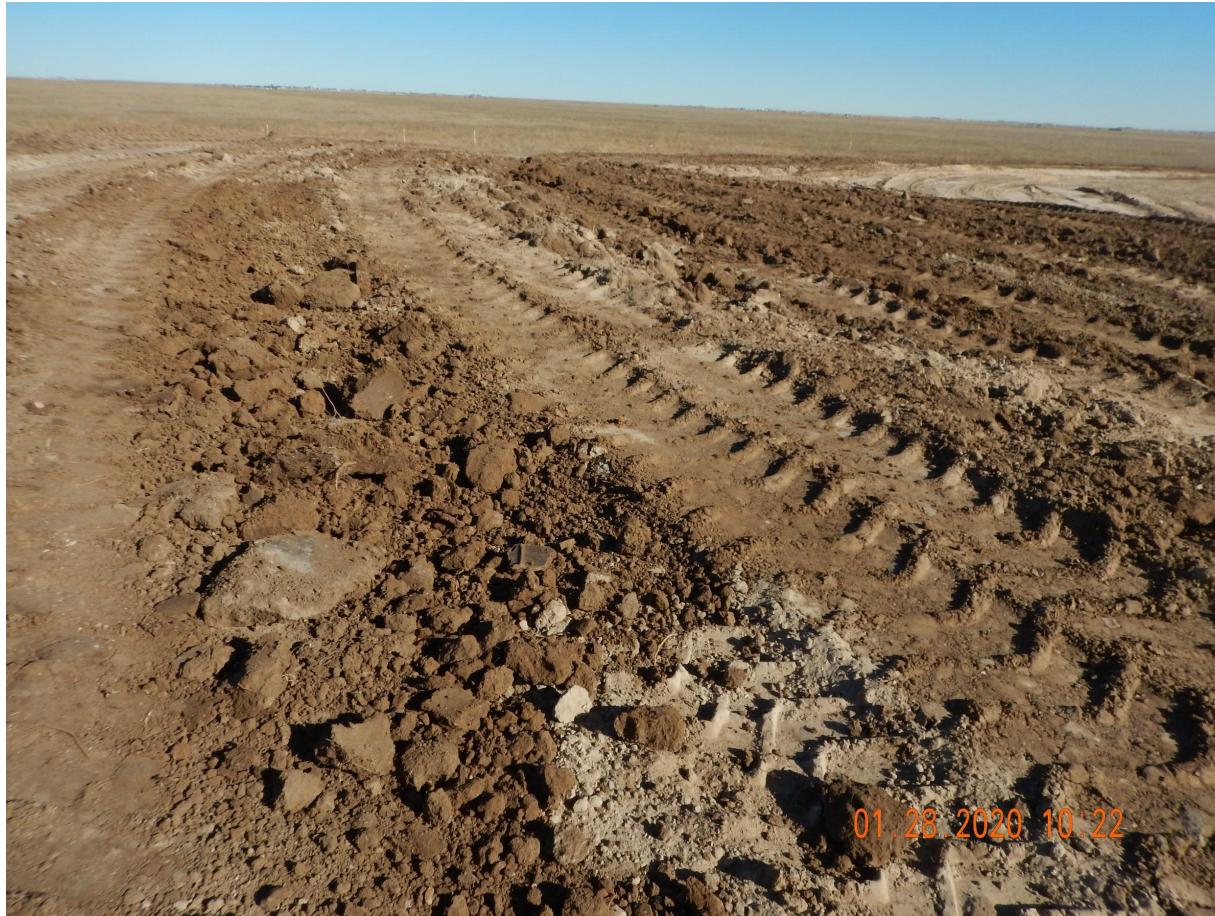
Photo 4. Photo taken from the topsoil stockpile, facing North. Photo illustrates there is some mixing of topsoil and subsoil. COGCC staff communicated to an Operator representative on location and on the phone, this observation and why topsoil should not be mixed.
