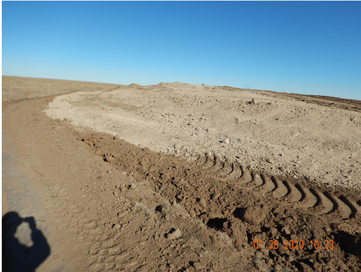
Photo 5. Photo taken from the west-facing topsoil stockpile, facing North. Photo illustrates subsoil being mixed with topsoil. COGCC staff communicated to an Operator representative on location and on the phone, this observation and why topsoil should not be mixed. Operator should remove any subsoil from the topsoil.
