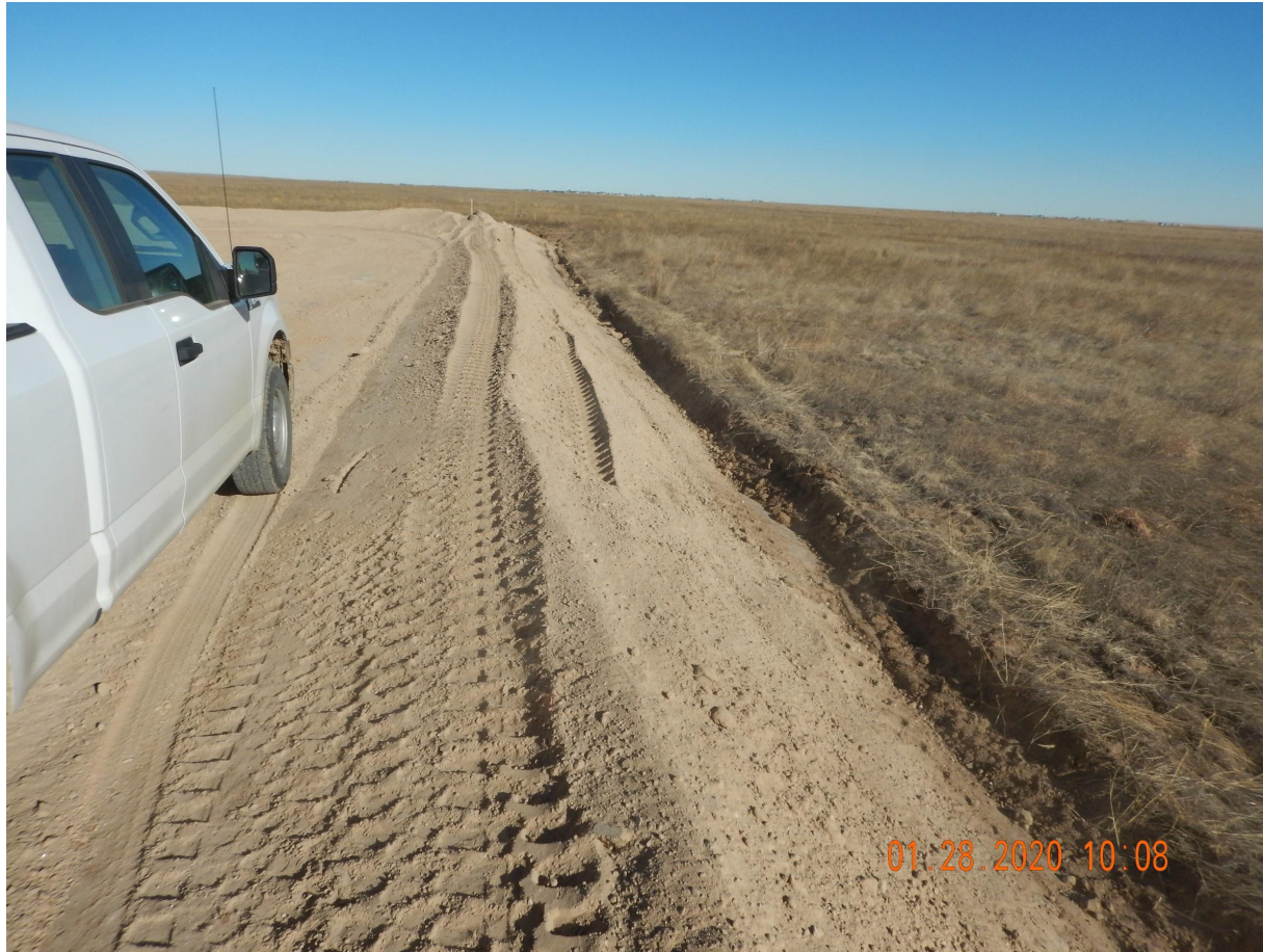
Photo 1. Photo taken from the northeastern perimeter of location, facing North. Photo illustrates a berm and ditch BMP. The ditch BMP could be installed to a greater depth and more “V” shaped.
