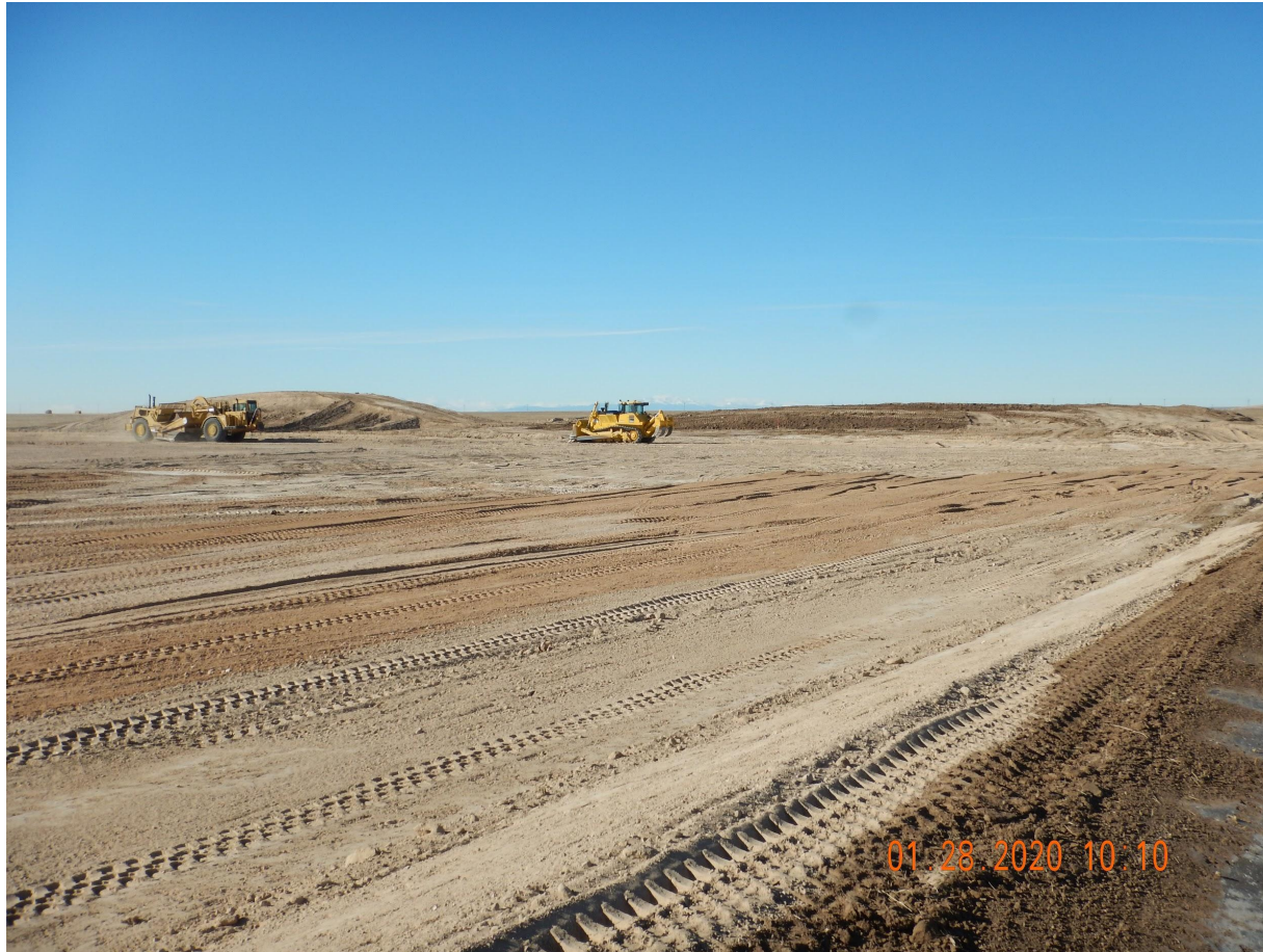
Photo 3. Photo taken from the northern perimeter of location, facing Southwest. Photo illustrates the stockpile to the right is topsoil and the stockpile to the left is of subsoil.
