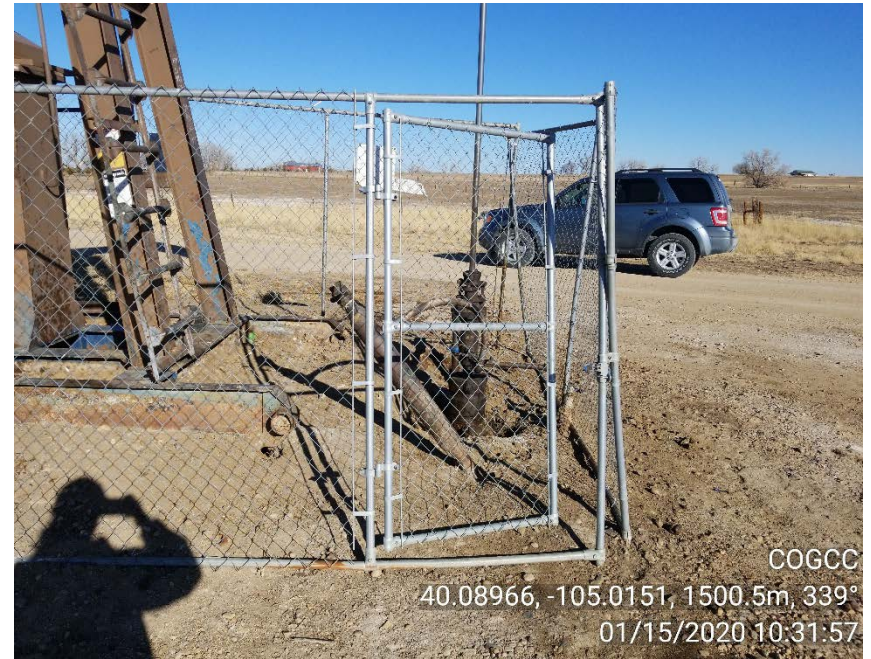
Photo 10 – Fencing around wellhead in disrepair
