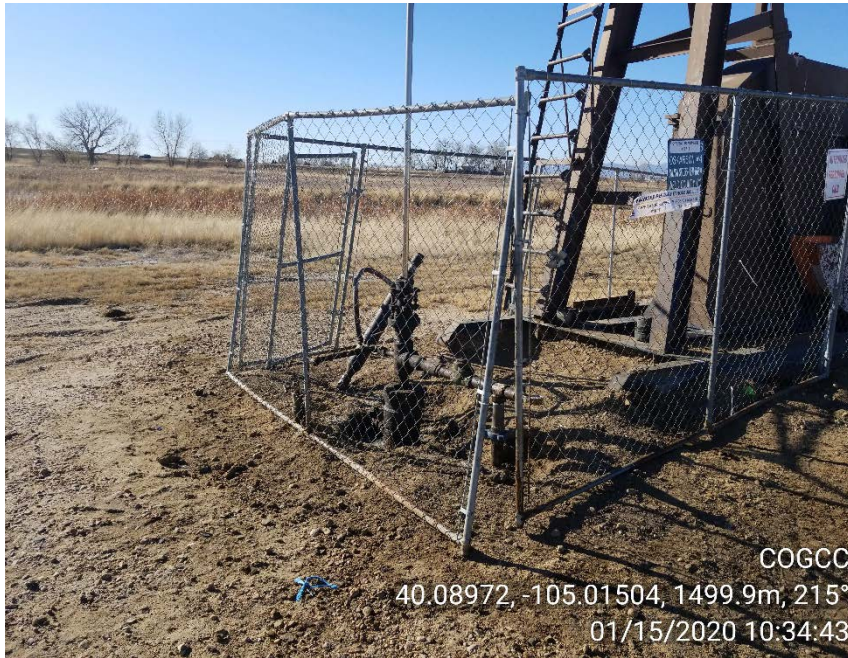
Photo 11 – Fencing around wellhead in disrepair
