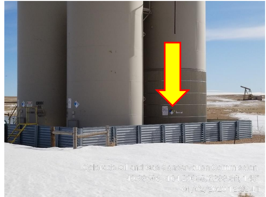
Photo 4 – Water Tank – Missing Content, Capacity and NFPA Labels
