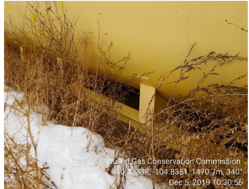
Photo 8: No containment surrounding tank.
