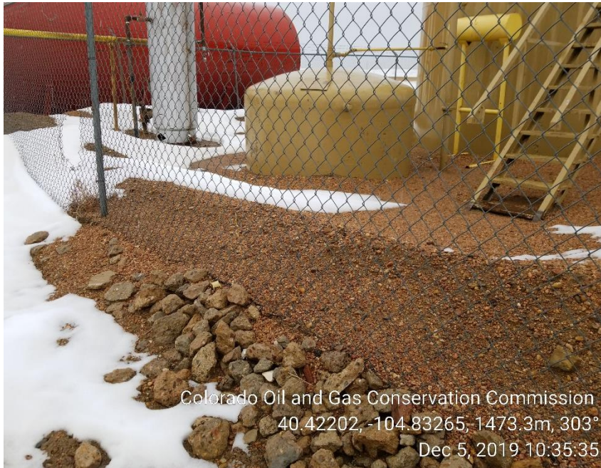
Photo 15: Inadequate berm
