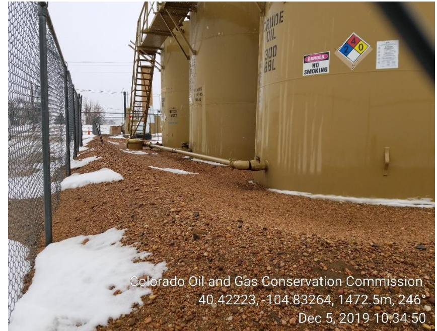
Photo 14: Inadequate berm
