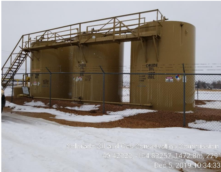
Photo 13: Tank Battery; INADEQUATE BERM
