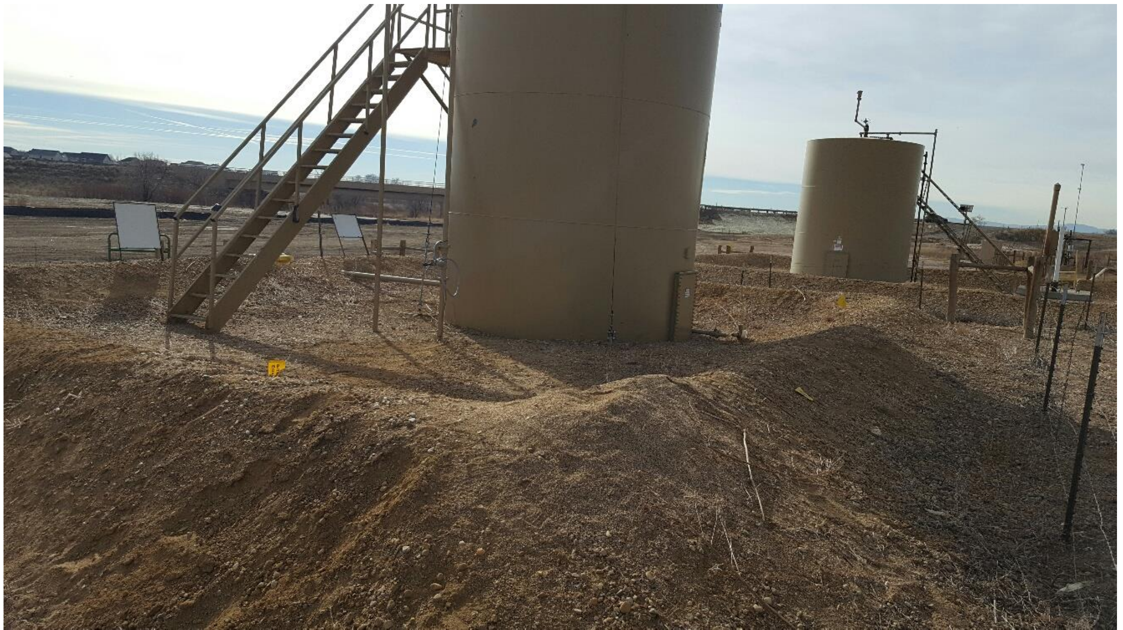
Figure #3 Tanks have been anchored down. Berms have been raised.
