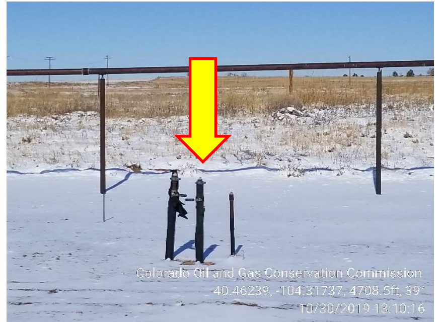
Photo 4 – Unmarked 1" Risers
