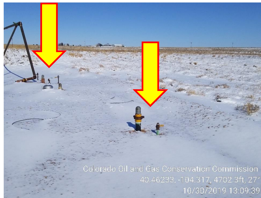
Photo 6 – Unmarked 1" and 3" Risers
