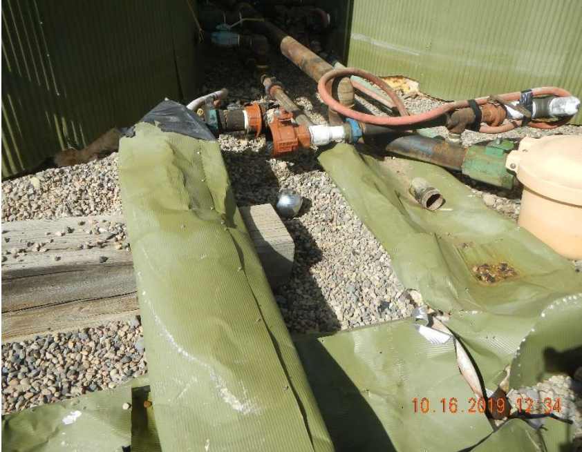
Photo #9 – View of the disassembled manifold where the spill/release occurred.
