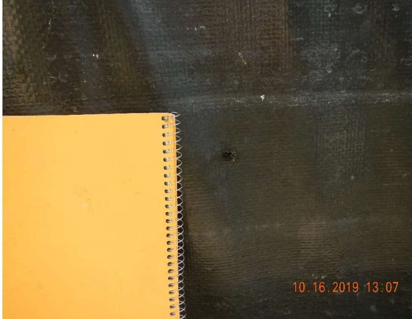
Photo #7 – View of a pen sized hole on the east side of the tank battery secondary containment liner.
