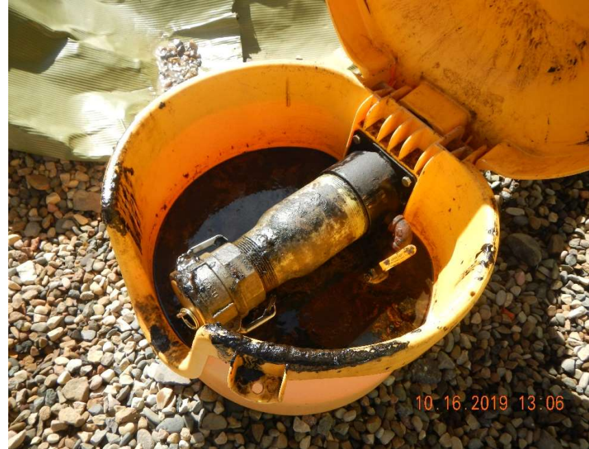
Photo #10 – View of the load out containment full of hydrocarbon fluids.
