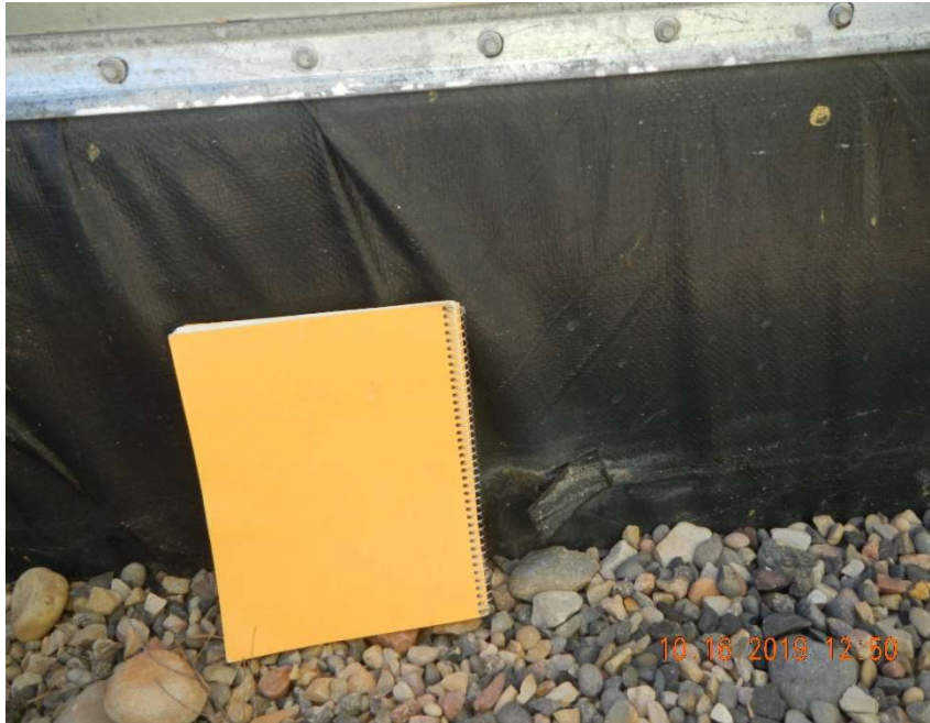
Photo #5 – View of a patch peeling off on the south side of the tank battery secondary containment liner.
