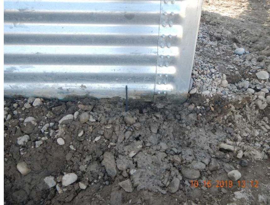
Photo #16 – View of fluids daylighting and hydrocarbon staining on the northwest corner of the tank battery
