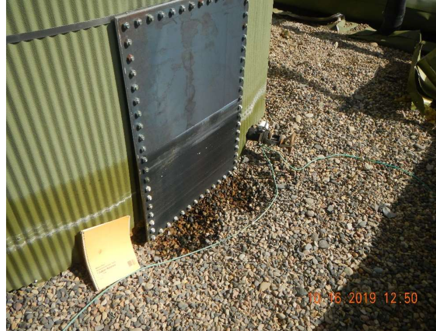
Photo #8 – View of the 10 inch and 20 inch bathtub line and the stained soil beneath man hatch on southeast 400 bbl condensate tank.
