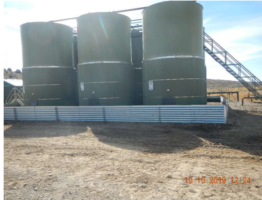
Photo #2 - View of the tank battery on location looking southwest. The tank battery consists of (2) 400 bbl condensate tanks, (3) 400 bbl produced water tanks and (1) unlabeled tank.
