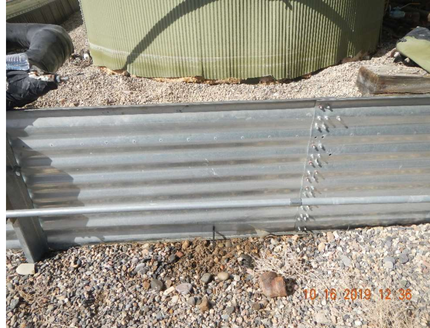
Photo #18 – View of moist soil on the east side of the tank battery. Photo was taken at the location of the hole in Photo 7.
