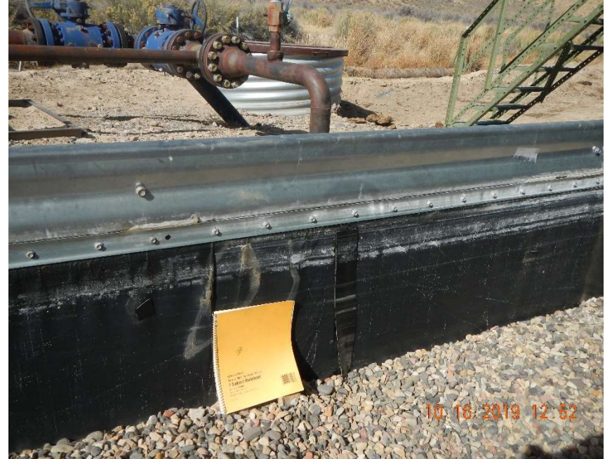
Photo #4 – View of patch peeling off on the west side of the tank battery secondary containment liner.
