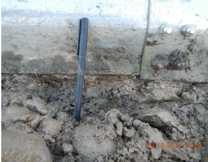
Photo #17 – View of fluids daylight on the northwest corner of the tank battery.
