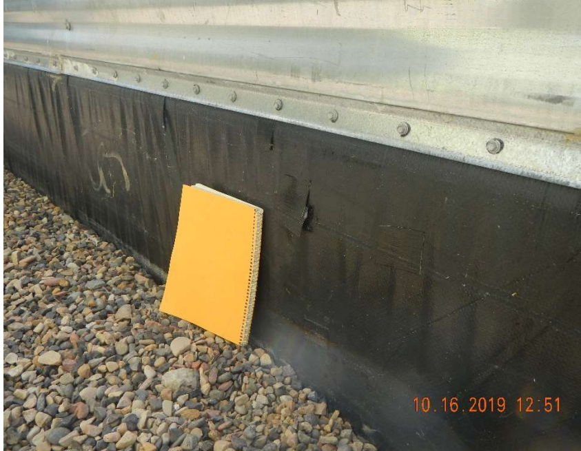
Photo #3 – View of multiple patches peeling off the secondary containment liner of the on the south side of the tank battery.
