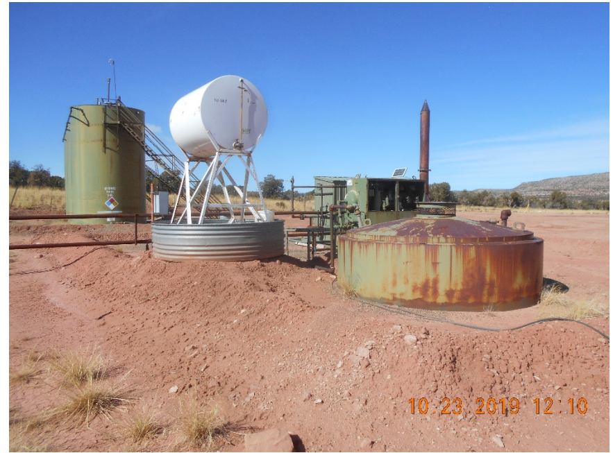
Chemical tank in secondary containment with improper/illegible labels.
