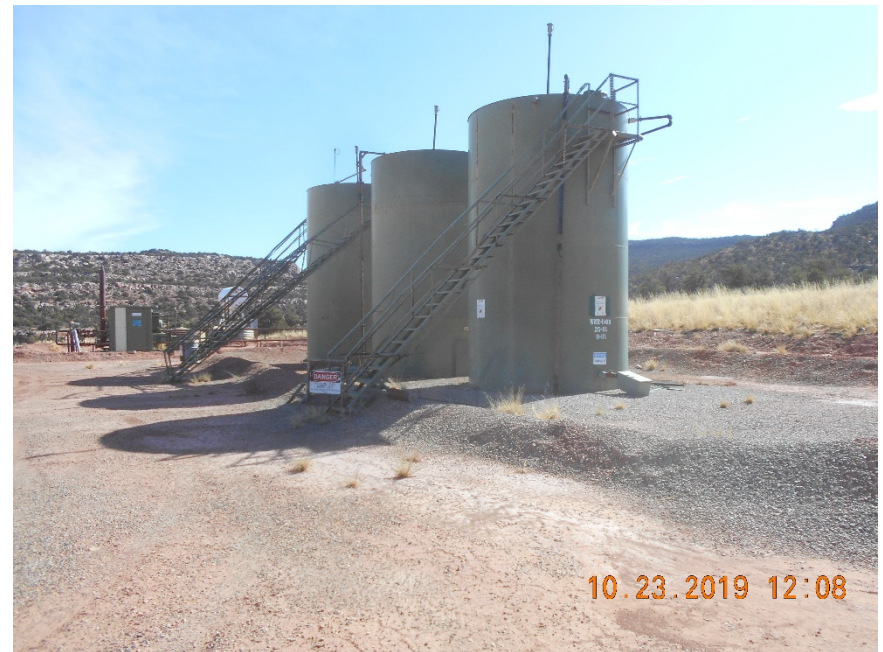
Tank Battery with unused catwalk section
