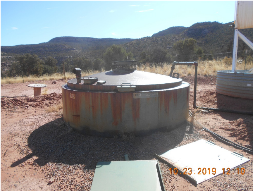
Blowdown tank with improper/illegible labels. Separator door panels in foreground.
