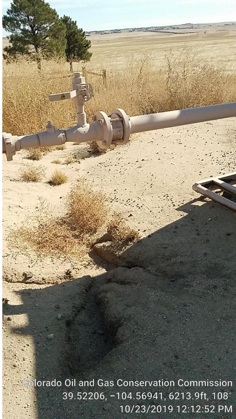
Erosion rill near gas meter run.
