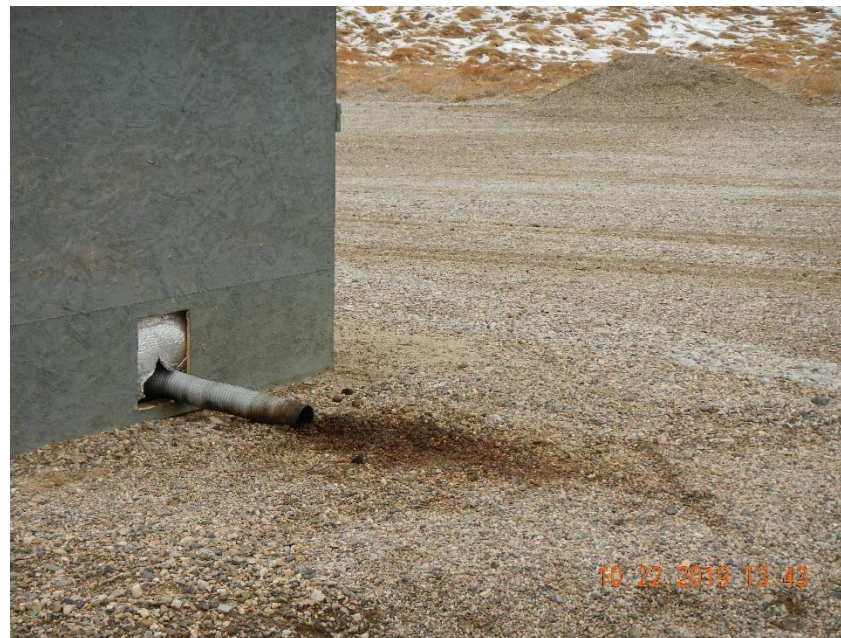
Photo 2. Stained soil at pump jack exhaust.
