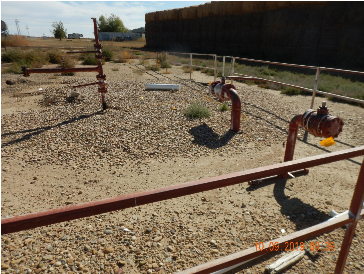
Photo 4. Photo taken from the tank battery location, facing East. Operator has failed to remove all equipment, remove gravel and perform final reclamation activities at the tank battery location.
