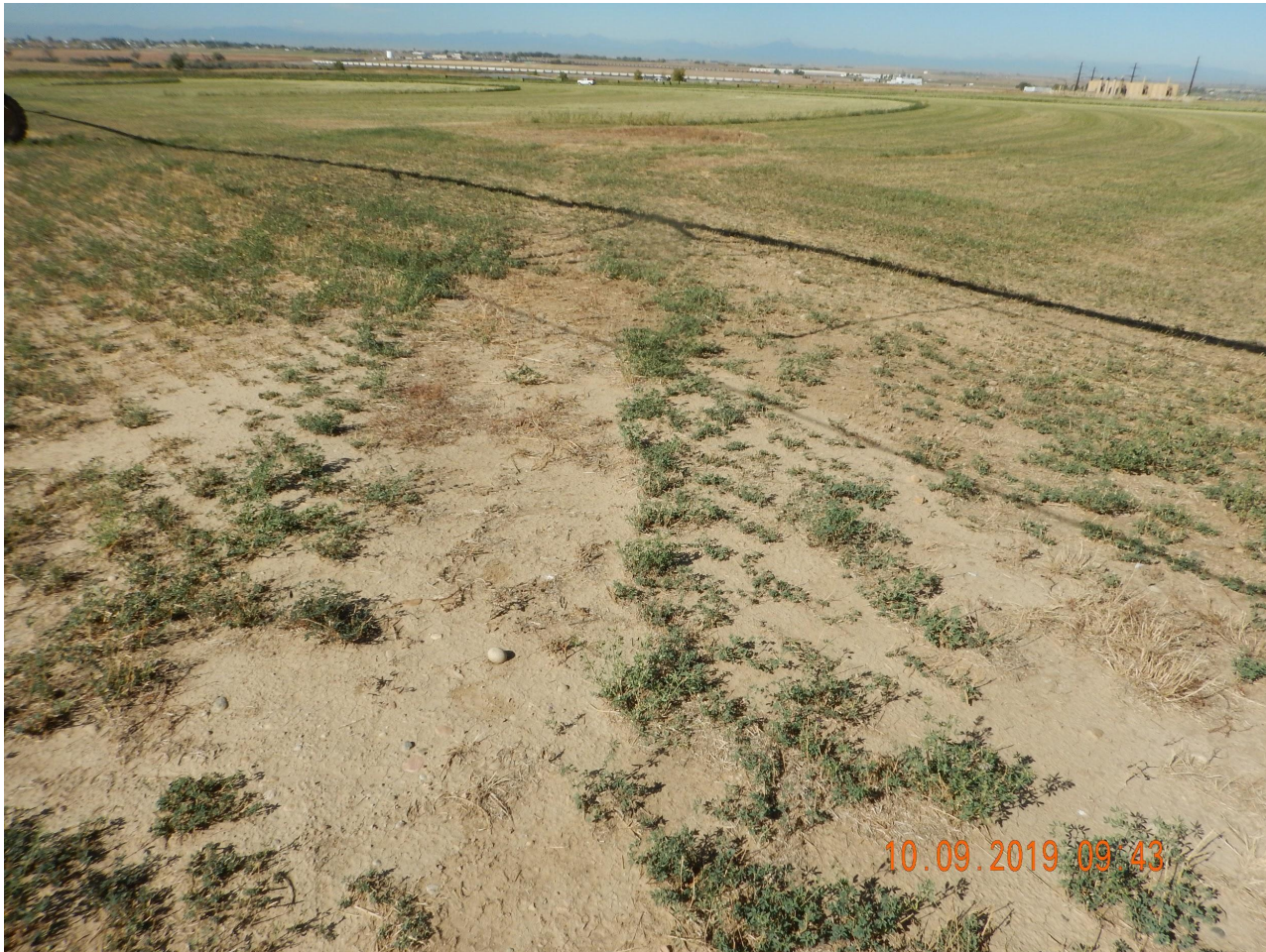
Photo 6. Photo taken from the well location access road, facing West. Photo illustrates the access road has not been properly recontoured and vegetation is not growing throughout portions.
