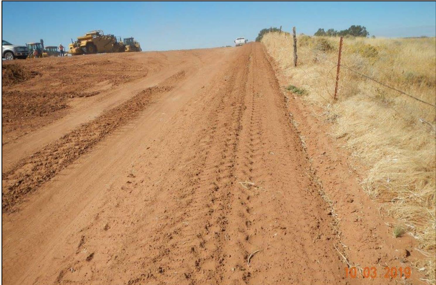
Photo 4. View of the northern portion of the project area facing westward. Ditch and berm are in place. However, loose soil on berms and in ditches is not stabilized and additional stabilization is needed.
