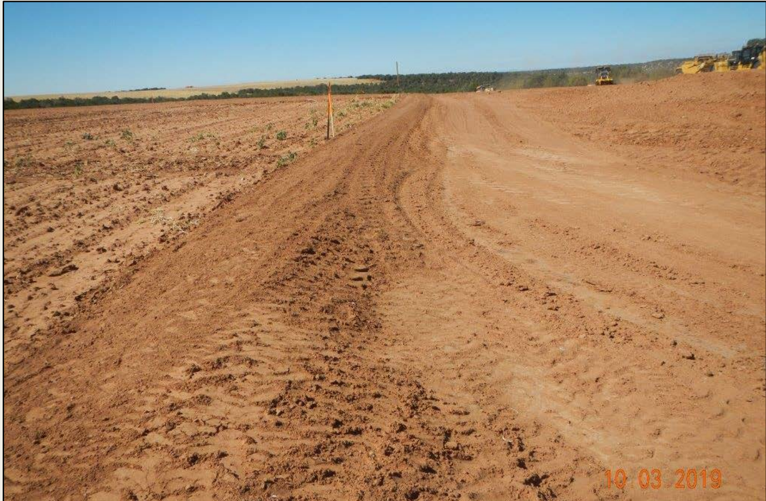
Photo 3. View of the southern edge of the project area from the southeastern corner facing westward. Ditch and berm in place. Loose soil on top of berm is not stabilized. Reference area on left side of photo is comprised of dryland crop field that is not planted at this time.
