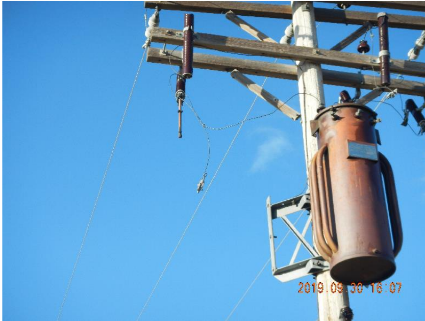
Photo 5: Power pole transformer and hanging disconnected jumper line.
