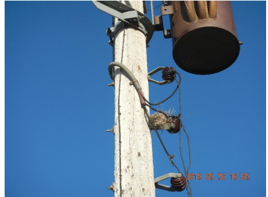
Photo 6: View of disconnected conduit line that has been bent towards the ground with lines hanging.
