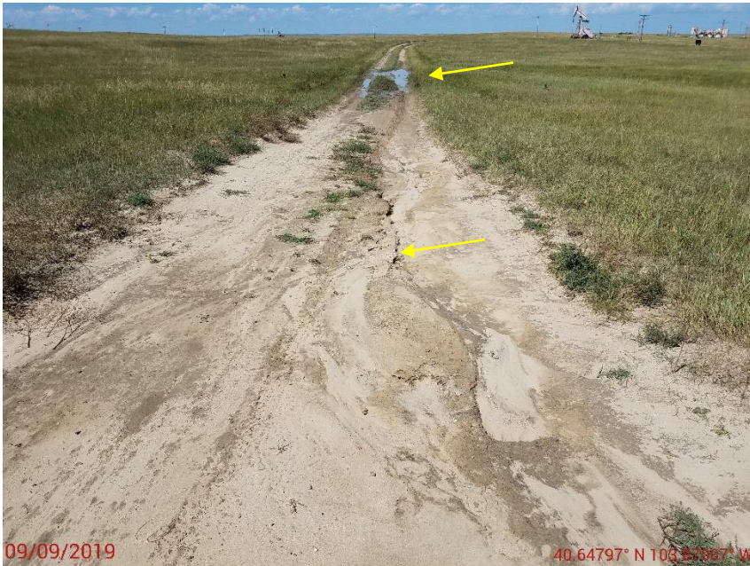
Photo 3: Photo shows stormwater erosion degradation on access road.
