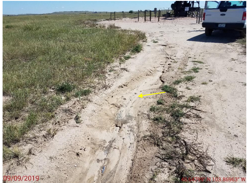
Photo 4: Photo shows stormwater erosion degradation on access road.
