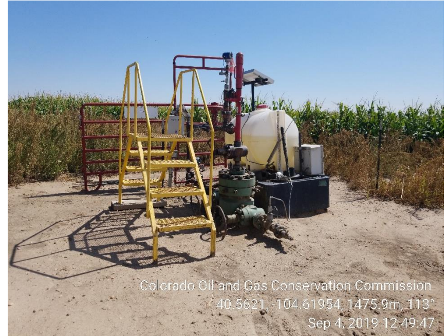
Photo 2: Wellhead w/methanol pump
