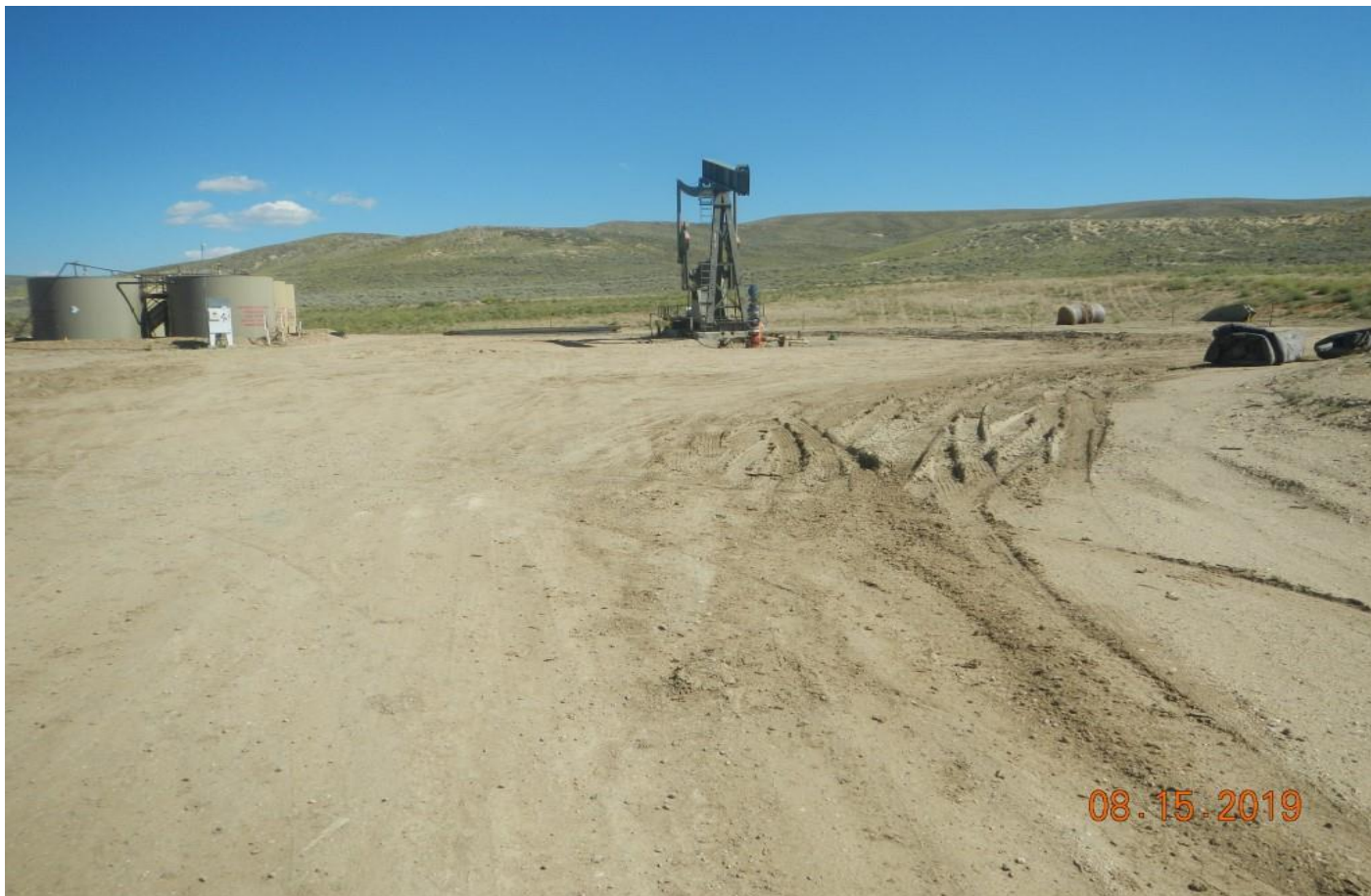
Photo#1: Overview of Location to East; unused equipment, rutting, debris.
