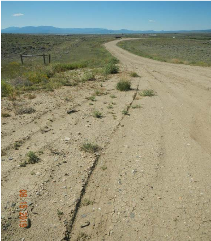
Photo#3: BMPs not installed along access road.
