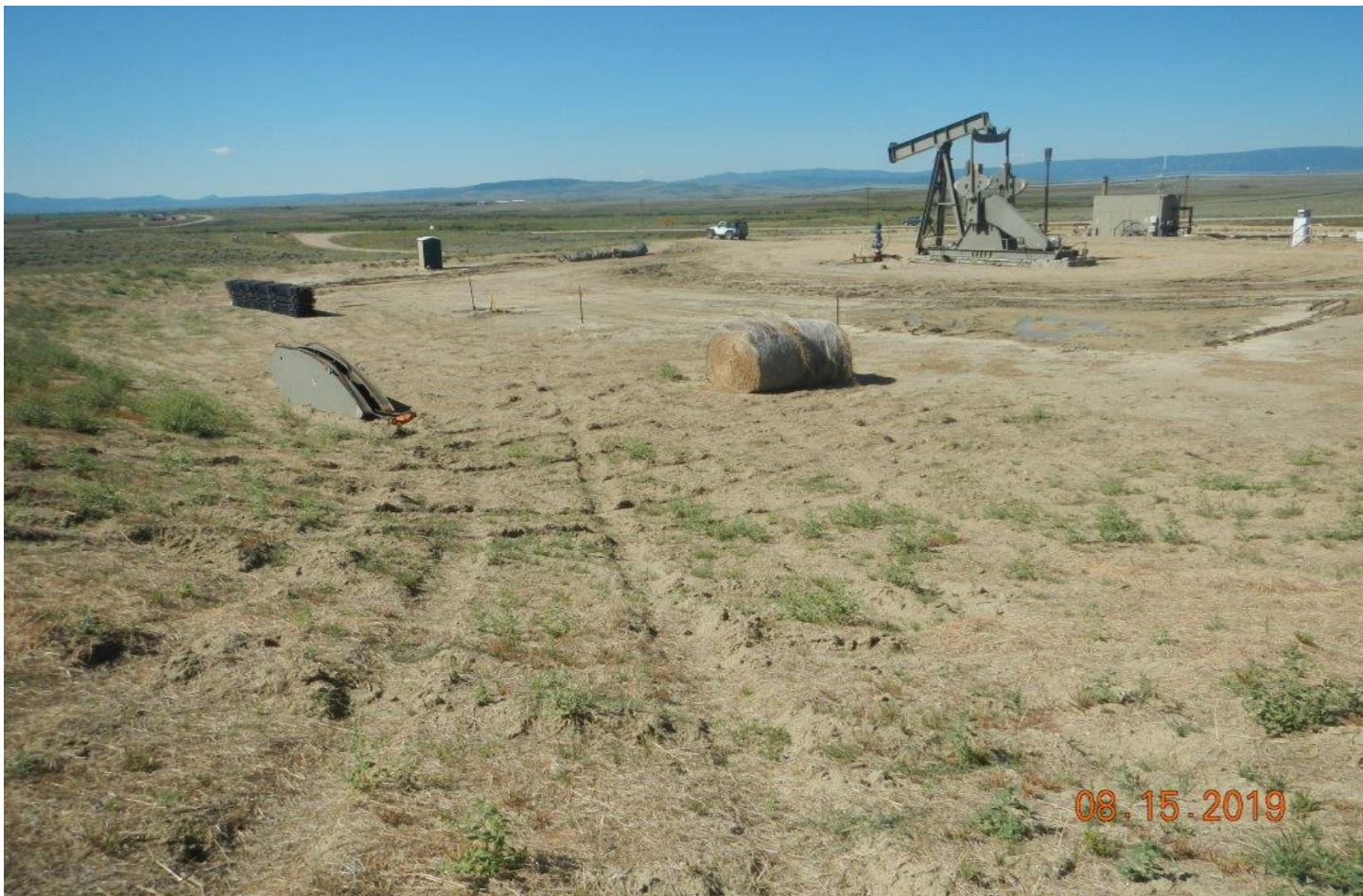
Photo#2: Overview of Location to Northwest; unused equipment, rutting, debris. .
