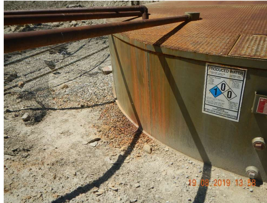
Photo #6 – Stained gravel and soil on the southeast side of the 95 bbl produced water tank.
