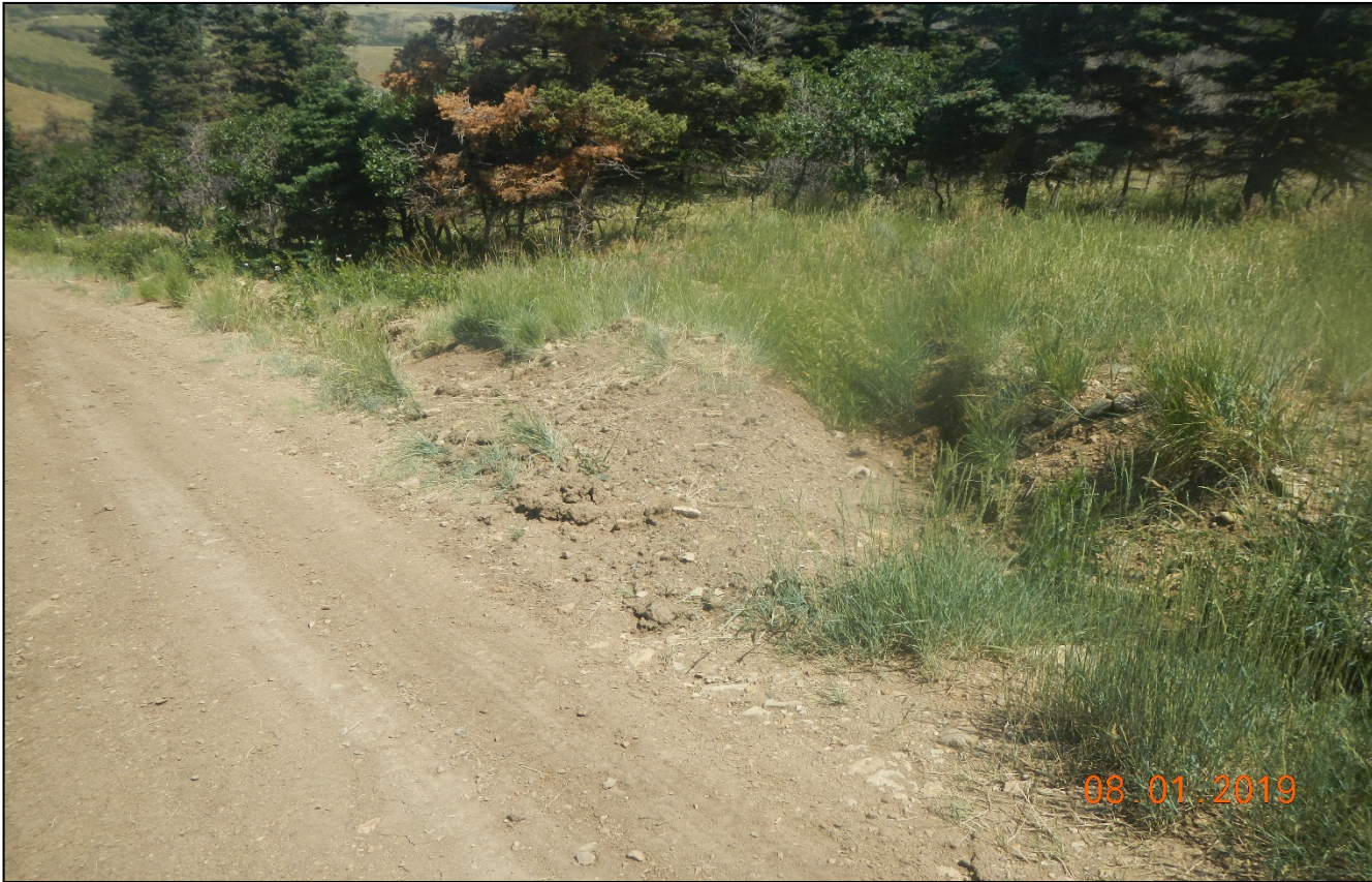
Photo 2. The road was graded and rock wattle damns were repaired. The sediment trap was cleaned out and erosion repaired.
