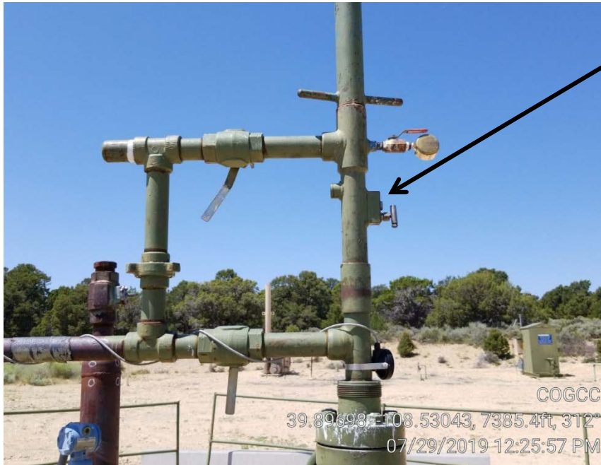
Photo 2. Well head gas leak.
