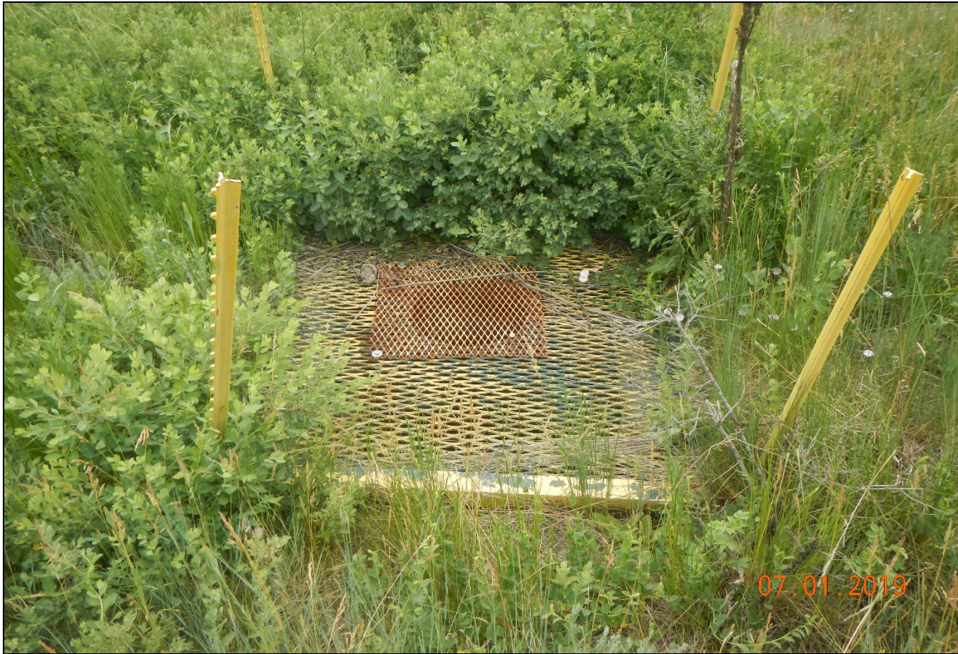
Photo 4. There is a hole with steel grate at center of location. Did not see conductor or casing in the hole.
