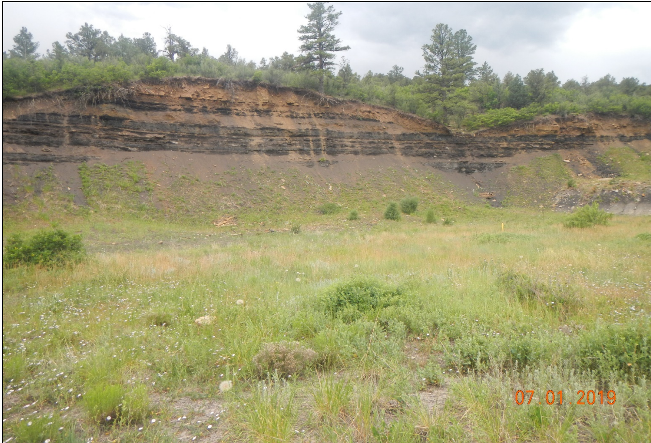
Photo 6. Facing toward the cutslope. The unstable cut slope is estimated to be 100 ft. high.
