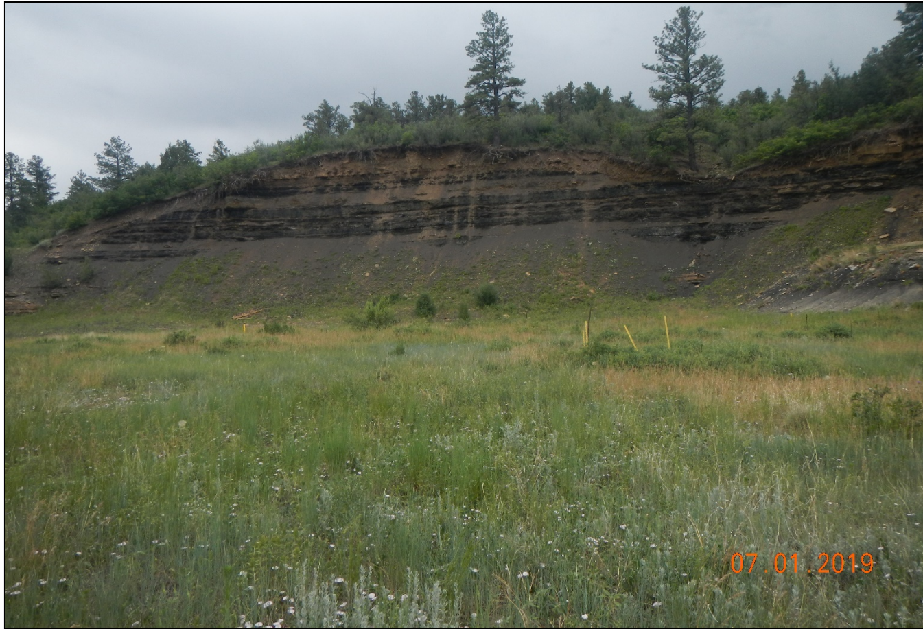
Photo 1. From the main road facing south toward the location. Unstable cut slope remains. Location not recontoured.
