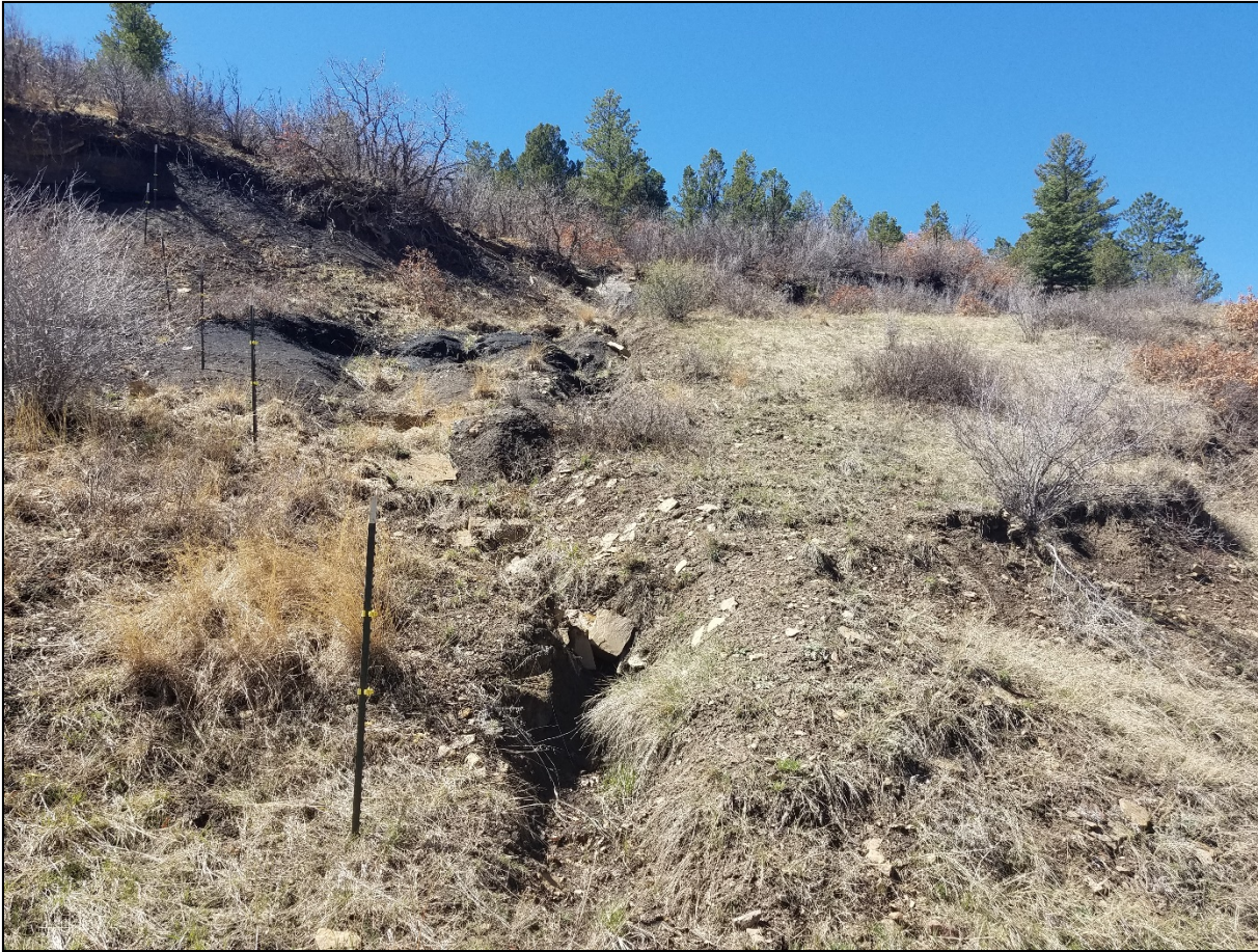
Photo 6. There is an erosion channel at the southwest cutslope.
