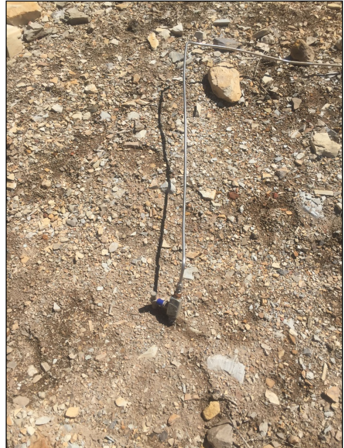
Process piping unprotected
