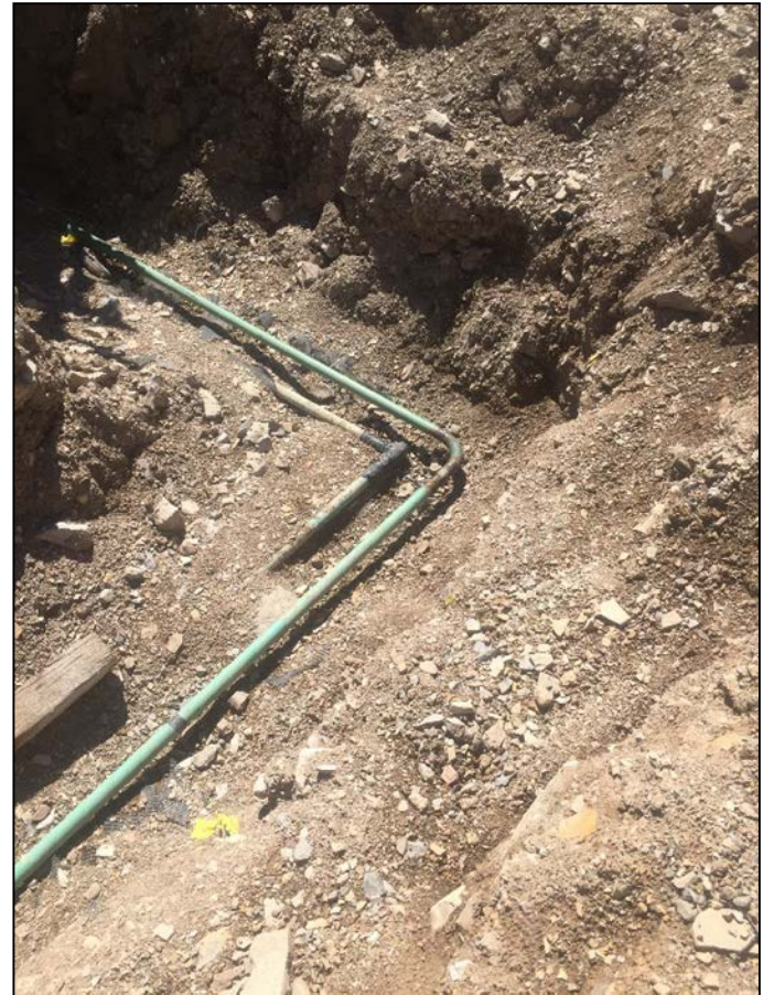
2" Dump line, Repairs made, target tee removed
