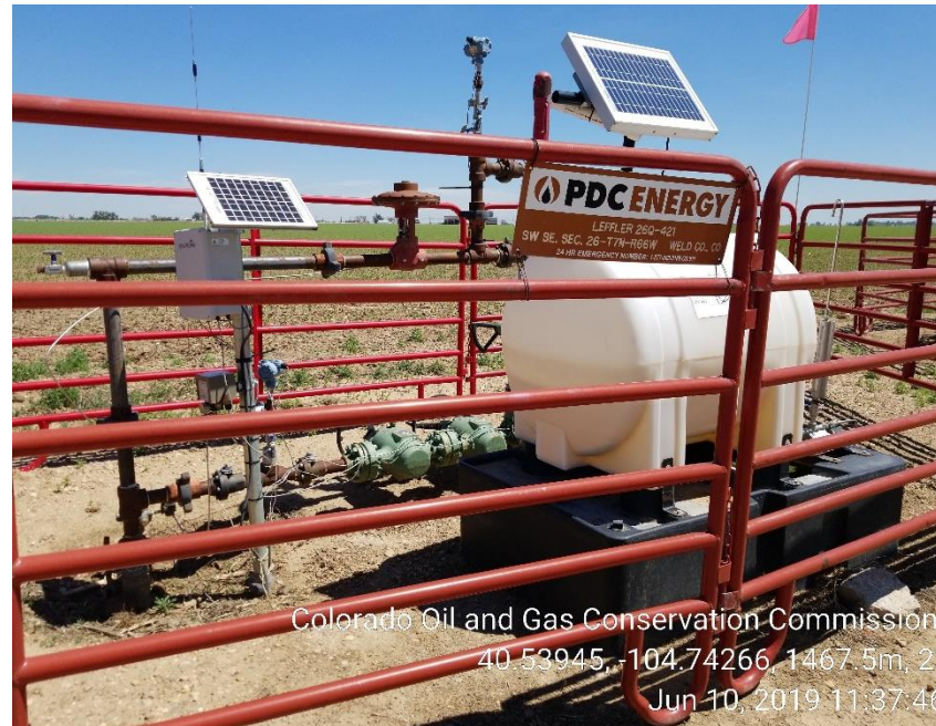
Photo 1: Wellhead with methanol pump
