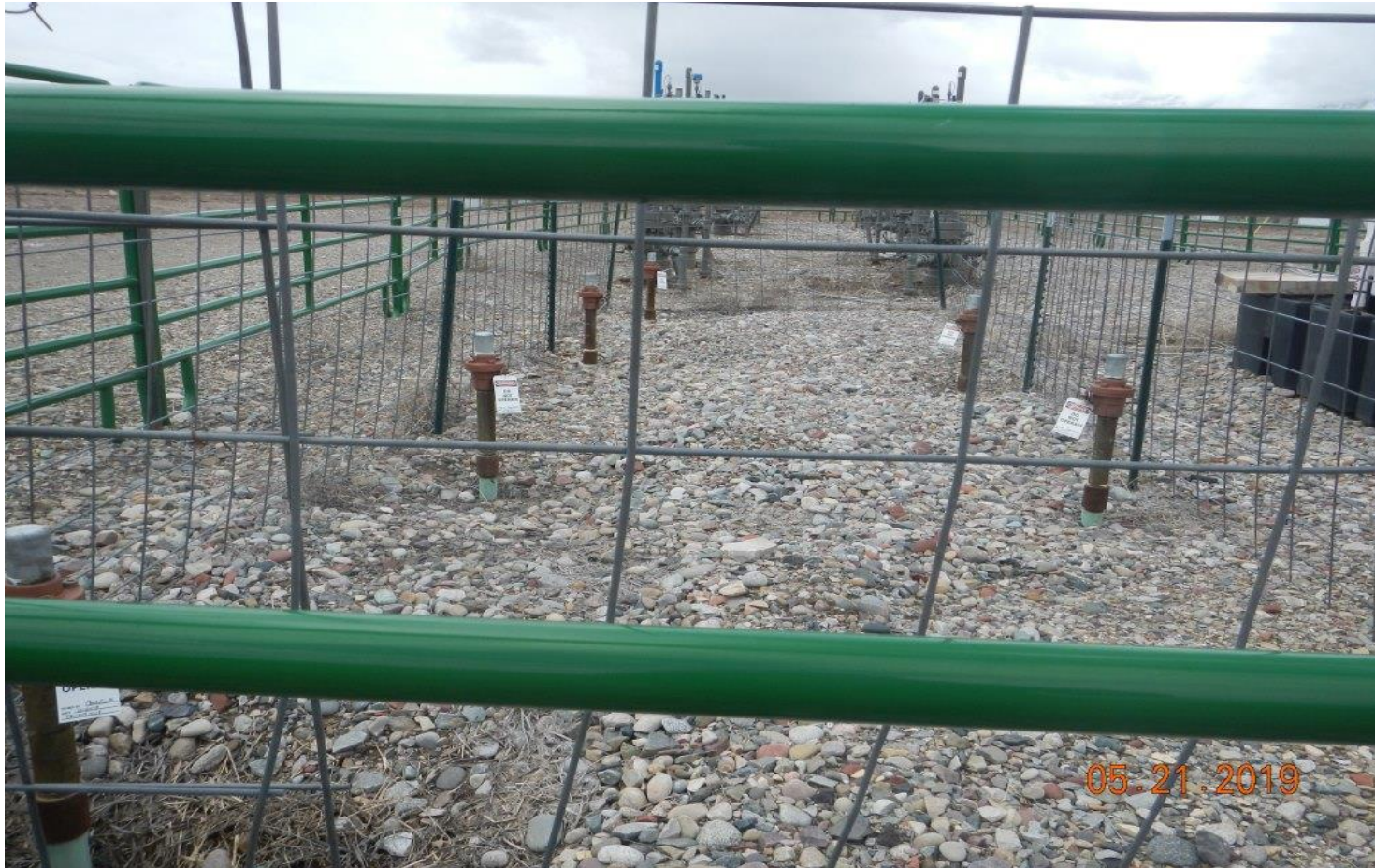
Photo#1: Six unknown risers at AL Well positions.
