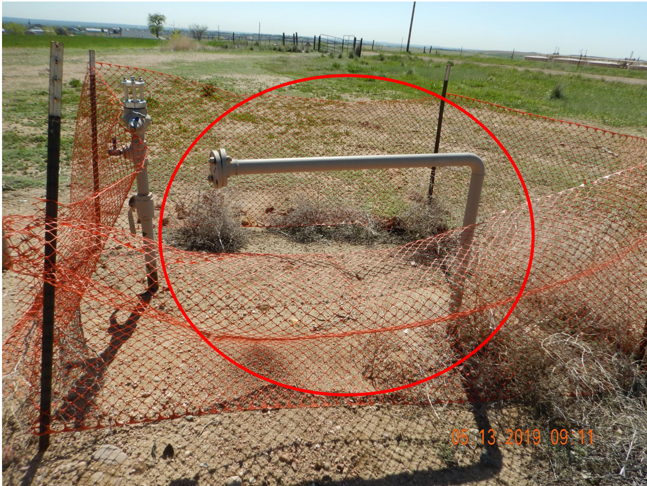
Photo 1. Photo taken from the tank battery location (39.972112, -104.924897), facing East. Riser (red circle) has been left on location. Operator shall remove riser per Rule 1004.a.
