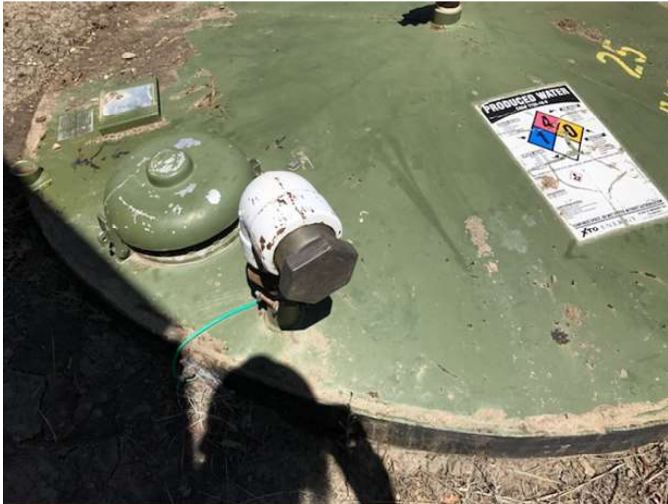
PHOTO 3: A (2) INCH BULL PLUG WAS INSTALLED INTO THE WATER TANK FITTING.
